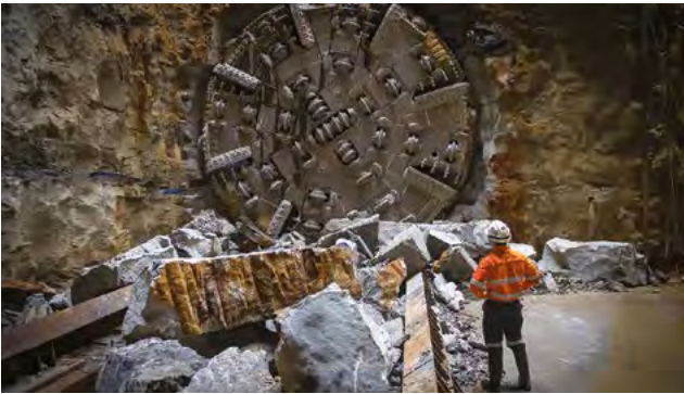
TBM Wendy breaking through at Blues Point on the Sydney Metro City & Southwest Project.
