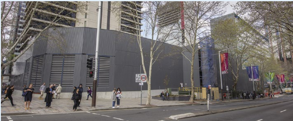
An acoustic shed used to minimise noise impacts on the Sydney Metro City & Southwest project.
