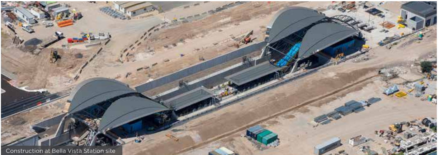
Construction at Bella Vista Station site
