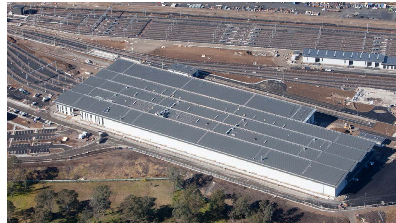
Construction taking place at Sydney Metro Trains Facility
