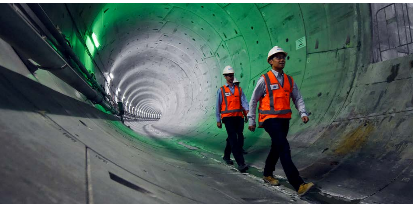
Workers inside a tunnel on the Northwest project
