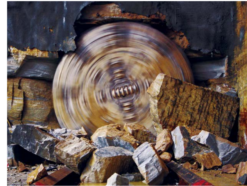
Tunnel Boring Machine breaking through at Showground Station
