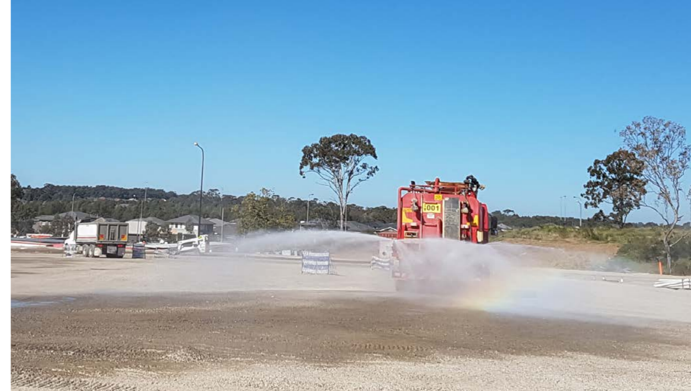
Water truck at Cudgegong Road Station site
