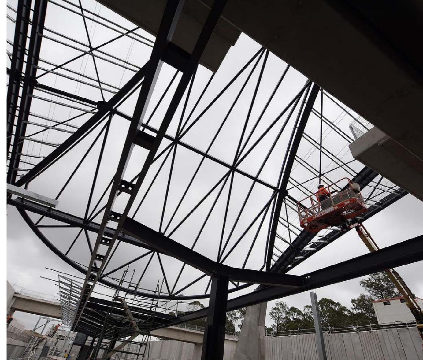
Workers assembling the canopy frames at Cudgegong Station
