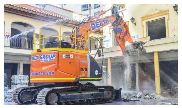
Figure 5: A Pulveriser being used for Demolition at the Victoria Cross Station Site
