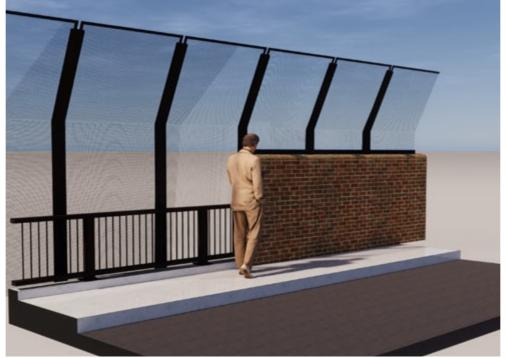
Figure 4.27 Typical vertical screen profile to Duntroon Street Bridge
