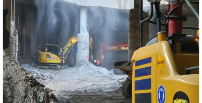
Misting system installed along the Metro Box.
