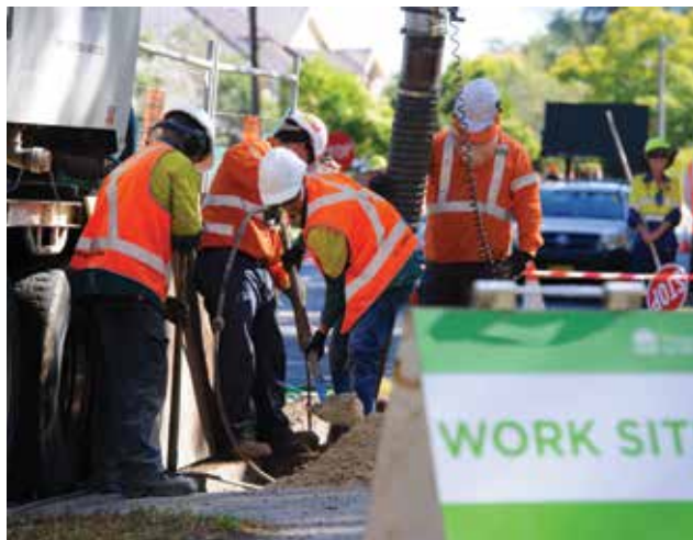
Potholing of buried services, Cherrybrook
