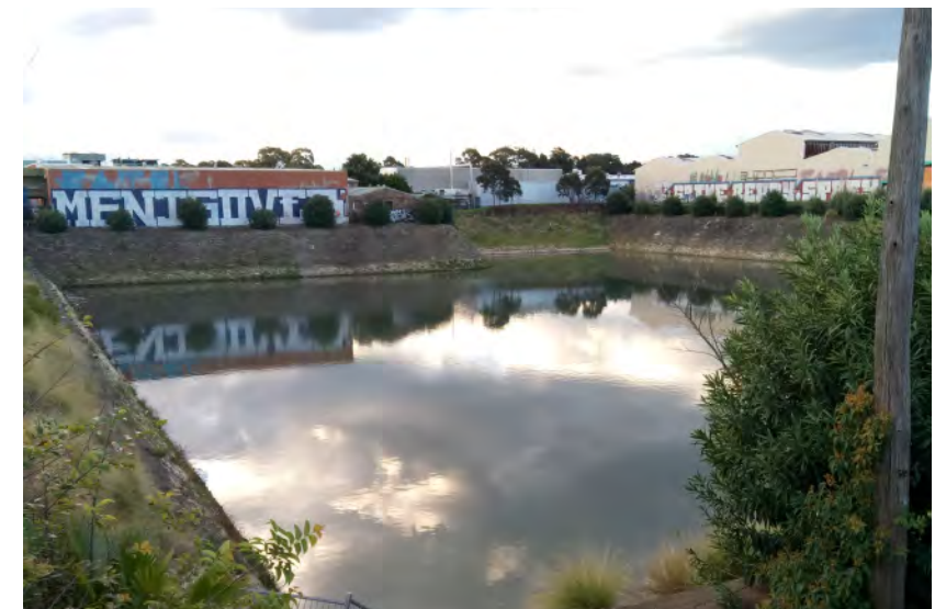
Sydenham Stormwater Storage Pit Source: COX/HASSELL
