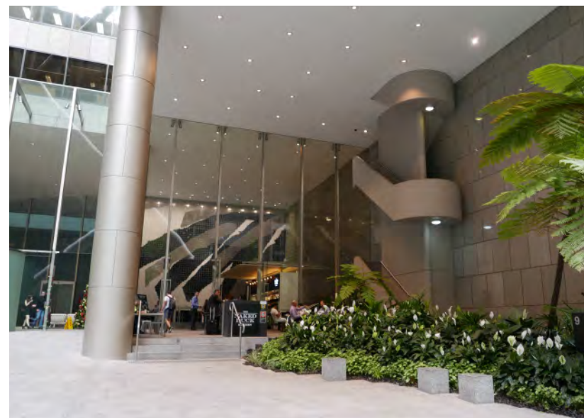
9 Castlereagh St, Sydney. The public domain is extended within the building’s site. Source: Cox Richardson
