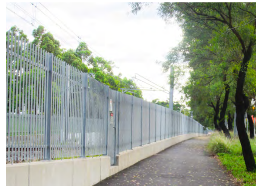
Homebush, Sydney. Rail corridor security fences should be robust, easily maintained, modular systems that are readily integrated with other urban design elements such as retaining walls. Source: AECOM.
