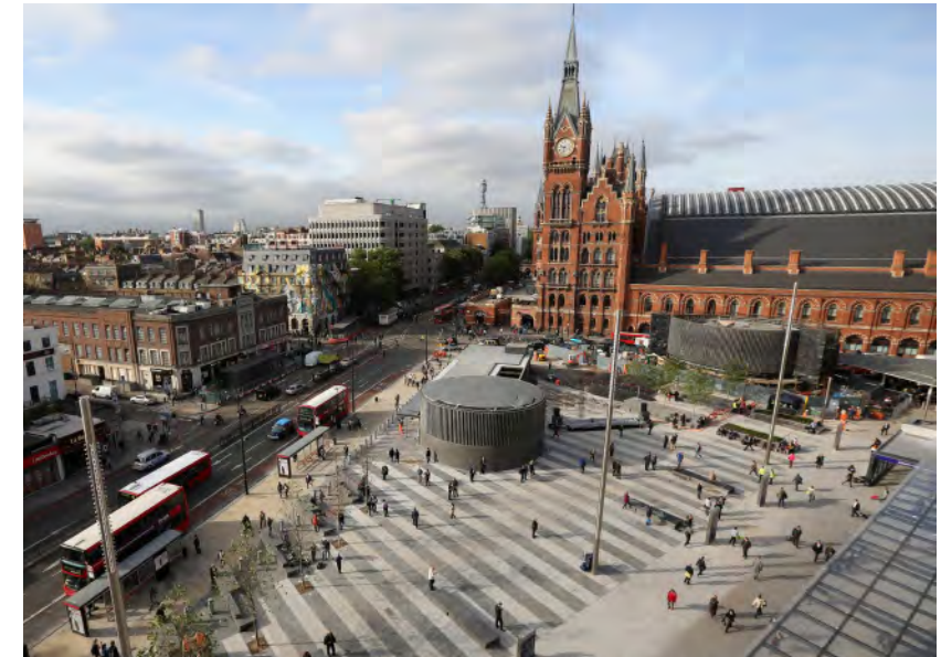
King's Cross Square, London. Good example of a well designed vent structure integrated with other functions within an urban setting Architect: Stanton Williams Source: Getty
