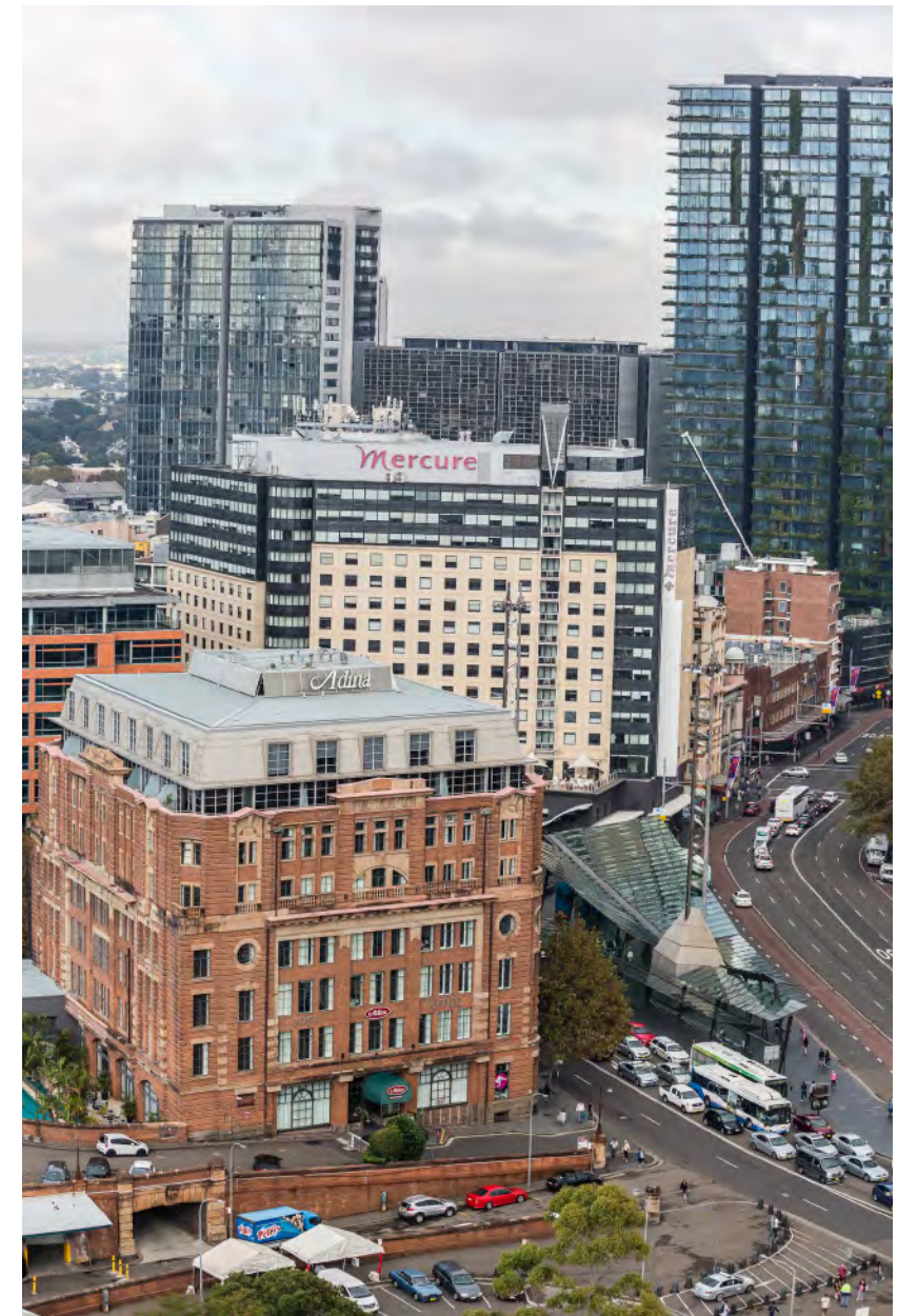
Central Station precinct. View over Railway Square looking south. Source: TfNSW
