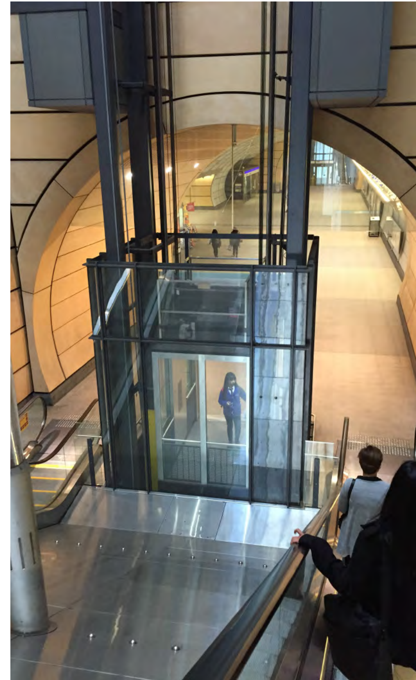
Macquarie Park Station, NSW. Glass sided lifts enable passive surveillance and sight lines through to the concourse. Architect: Hassell Source: Cox Richardson
