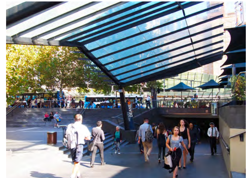
Design paths and ramps for access for all. All modal connections must be located in convenient, safe, well-lit areas with good natural surveillance. Source: AECOM.
