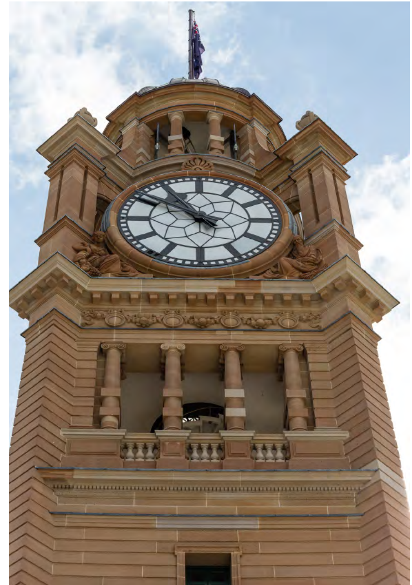
Central Station Clock Tower Source: TfNSW
