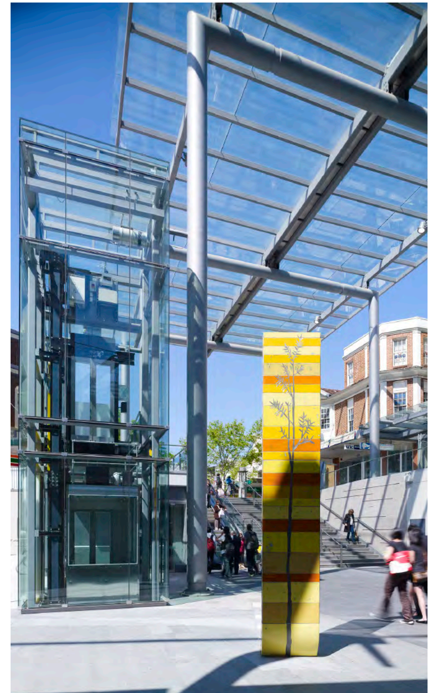
Chatswood Transport Interchange, NSW. Good example of a glazed lift and shaft Architect: CoxDesignInc. Source: Cox Richardson
