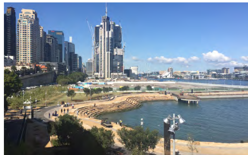
Barangaroo South under construction & Headland Park Source: Cox Richardson
