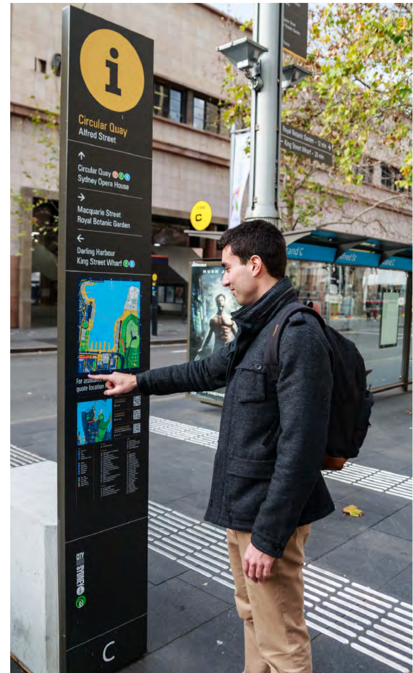
Circular Quay, Sydney. Signage and wayfinding enables clear sightlines of the interchange precinct. Source: TfNSW
