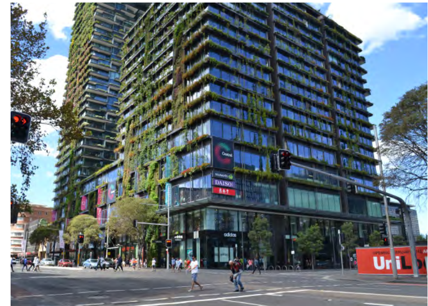
Central Park, Sydney. Landscaped facade treatment helps cool the microclimate. Architect: Jean Nouvel Source: Cox Richardson
