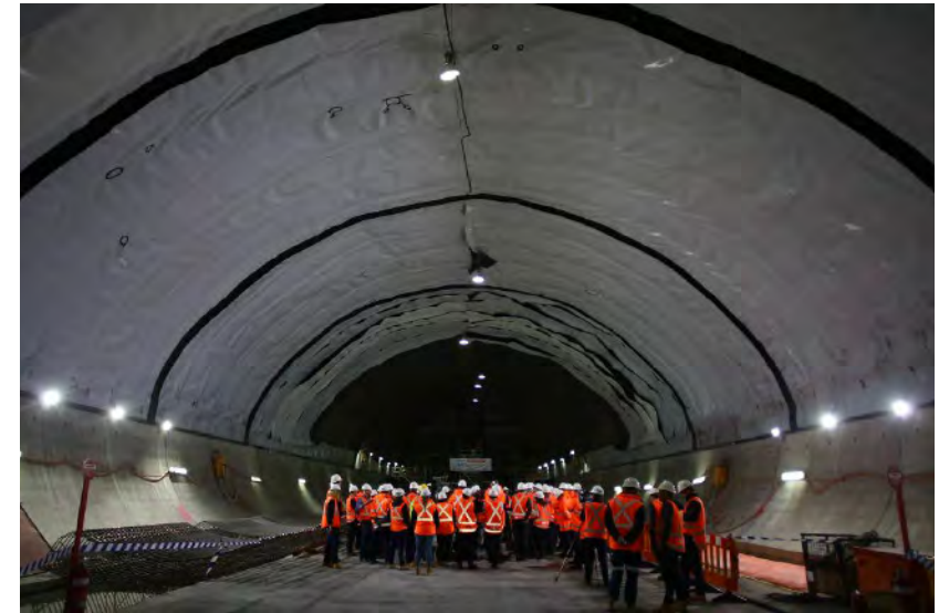
Construction of Sydney Metro Northwest. Source: TfNSW
