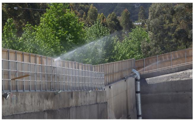
Figure 11 - Dust Mitigation at Norwest Station Site
