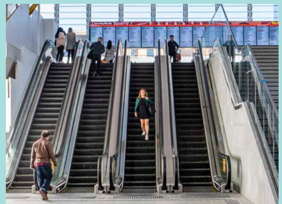
New escalators at Central.
