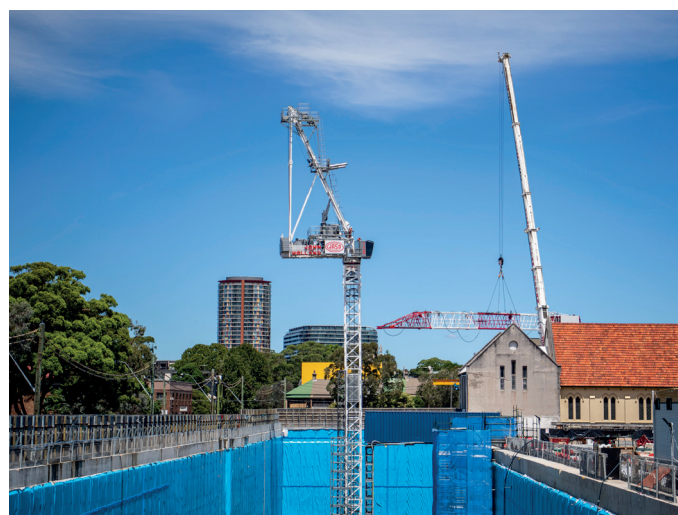
The tower cranes have been doing the heavy lifting inside the Waterloo station box
