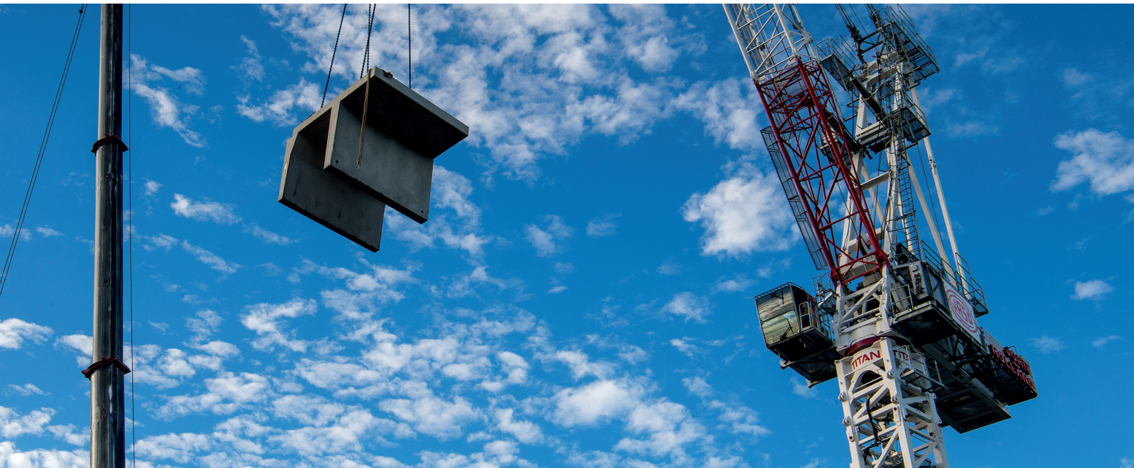
Precast elements lifted into the box to build the future station platforms
