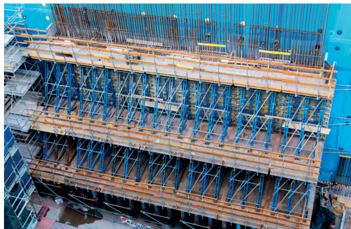
The A-frame formwork is higher than standard at 10 metres tall
