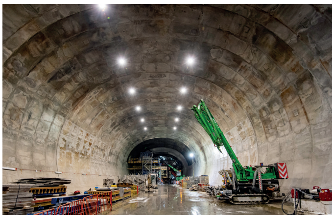
Formwork, waterproofing and concrete lining is nearing completion in the Victoria Cross station cavern
