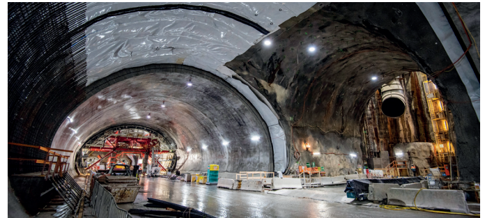
Formwork, waterproofing and concrete lining underway at Barangaroo
