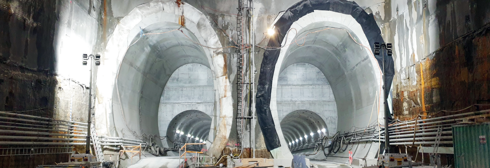
The tunnel portals (nozzles) inside the Crows Nest station box
