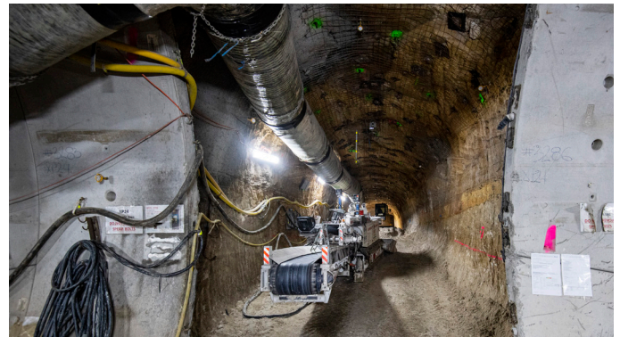
Excavation of a cross passage
