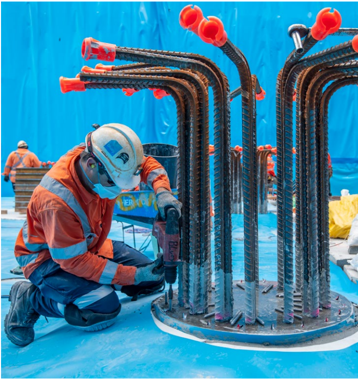
A worker drills bolts to secure the top of the pile.
