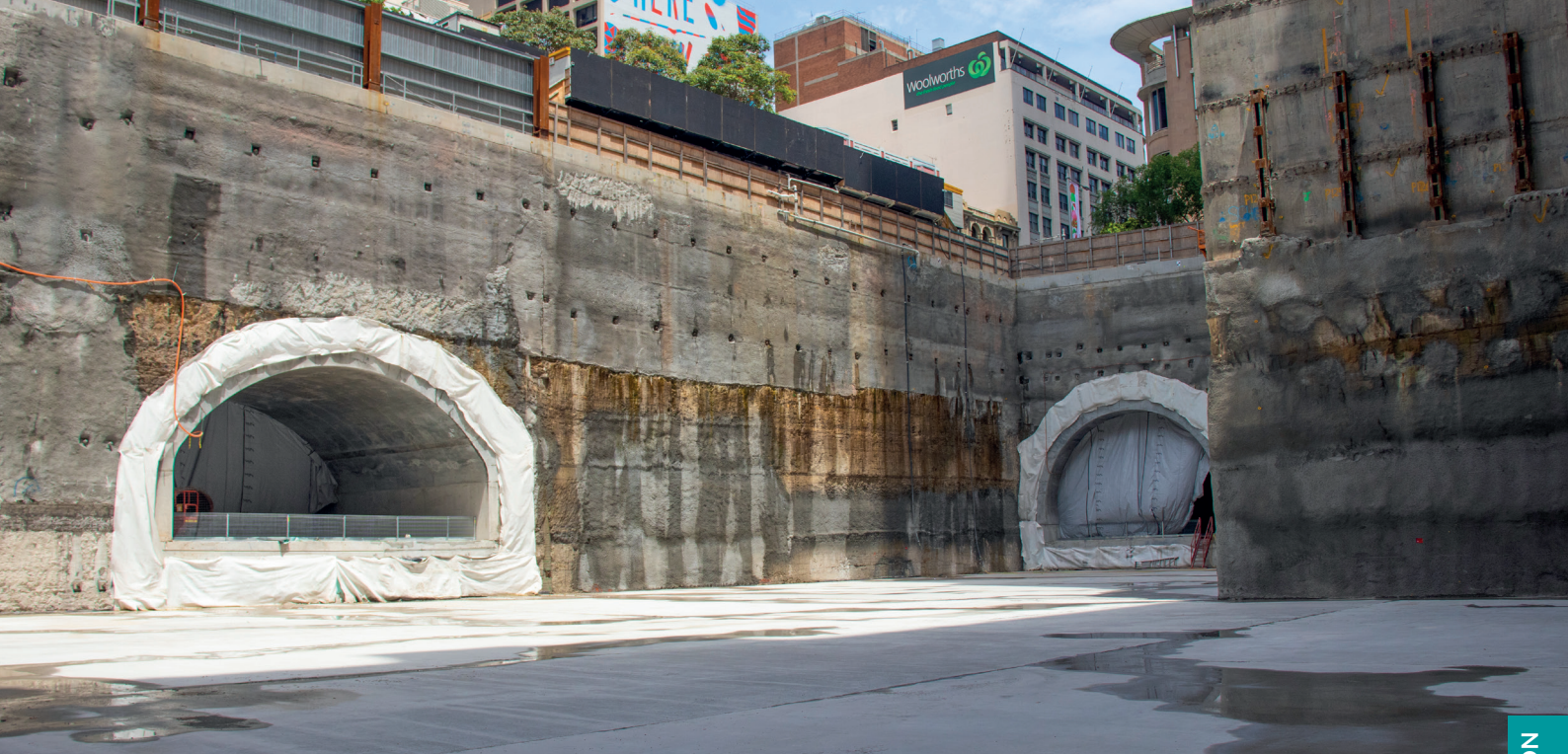
The Pitt Street North shaft is now complete and ready for hand over to the follow on contractor
