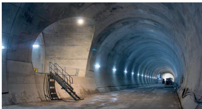
One of the twin underground station caverns beneath Castlereagh Street where the future Sydney Metro trains will pick up and drop off passengers
