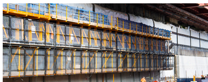
The innovative self climbing scaffold system used to construct the perimeter walls of the station box
