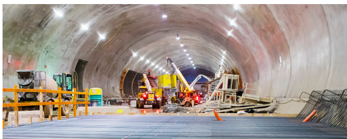
Over 2,500 tonnes of steel will be used to form the permanent structures inside the Barangaroo crossover cavern
