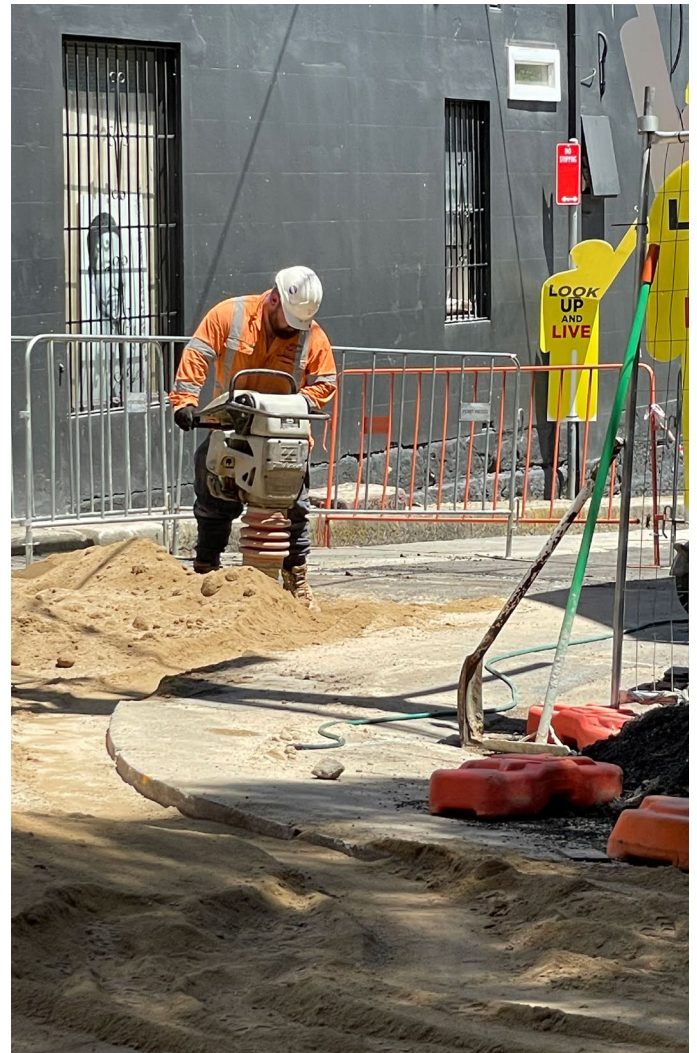
Compacting the ground at the corner of Albion Way and Bellevue Street.
