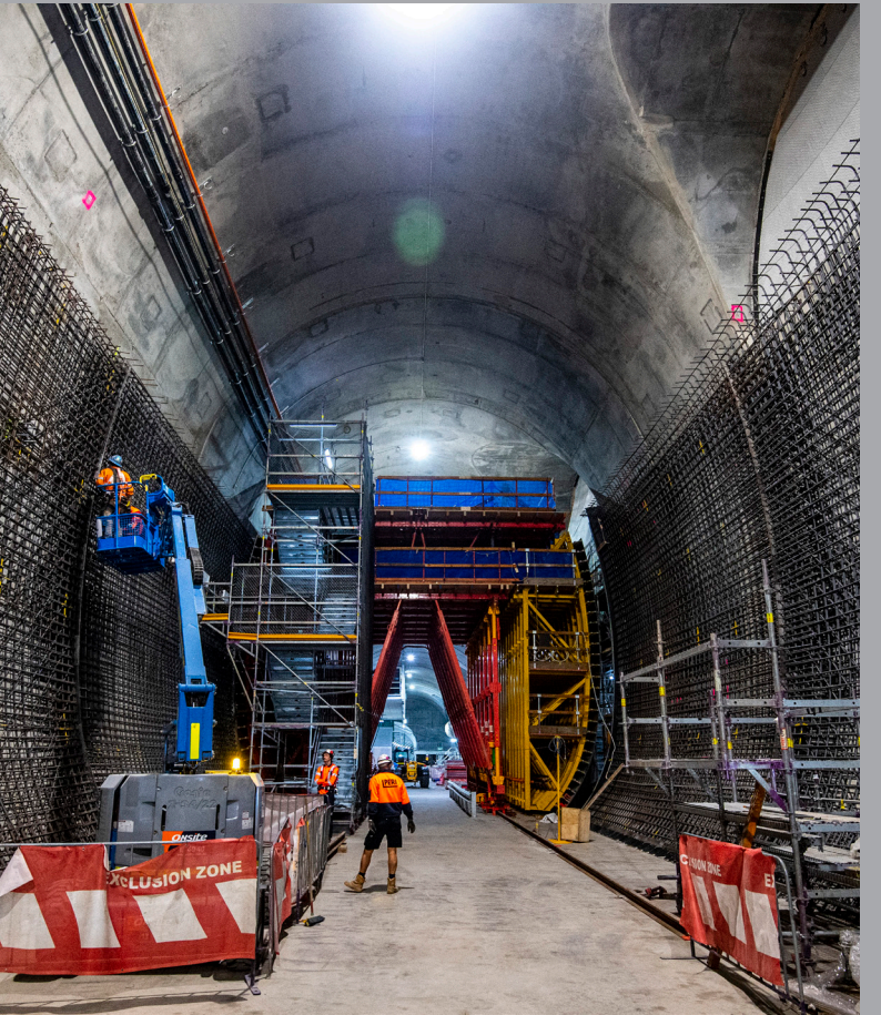
Wall reinforcement work underneath Castlereagh Street
