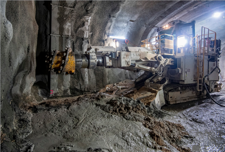
Matilda cutting through sandstone under 50 Martin Place
