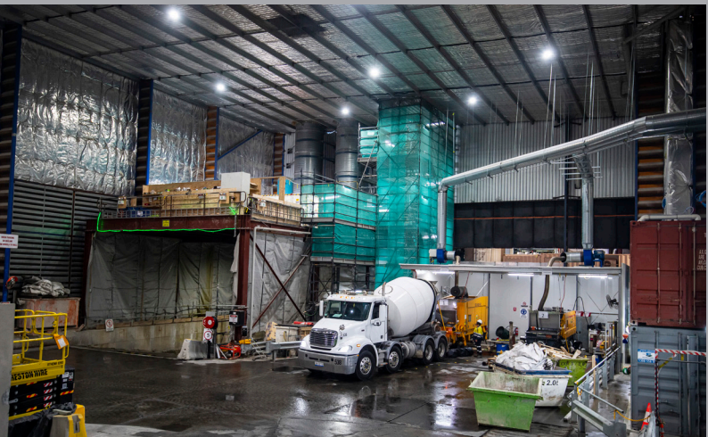
Concrete pumping station at Bligh Street site
