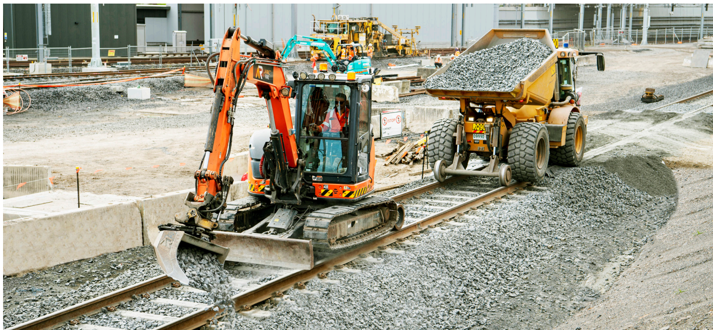
More than 15,000 tonnes of rock ballast is being used in the expansion of the Sydney Metro Trains Facility at Rouse Hill.
