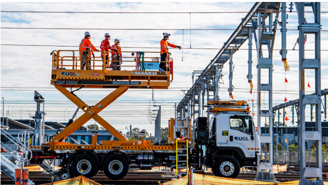
Our team is installing the wiring needed to power the new trains.
