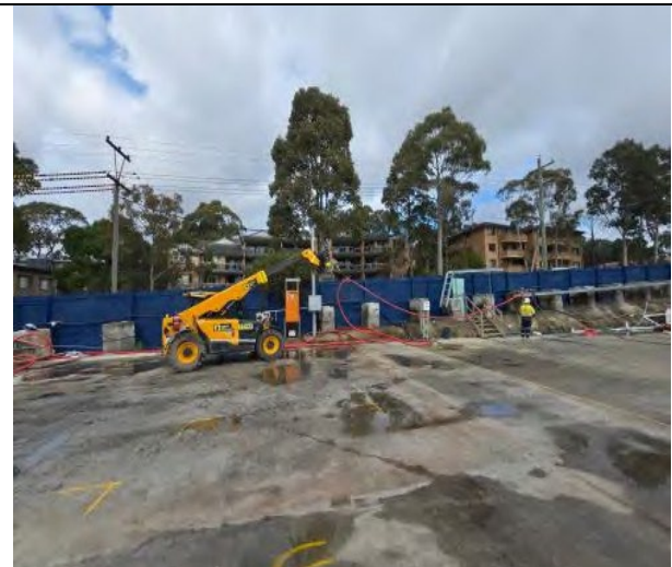
Figure 2.10–Westmead: Hoarding defect rectification works adjacent to Bailey Street commenced, with removal /relocation of services.
