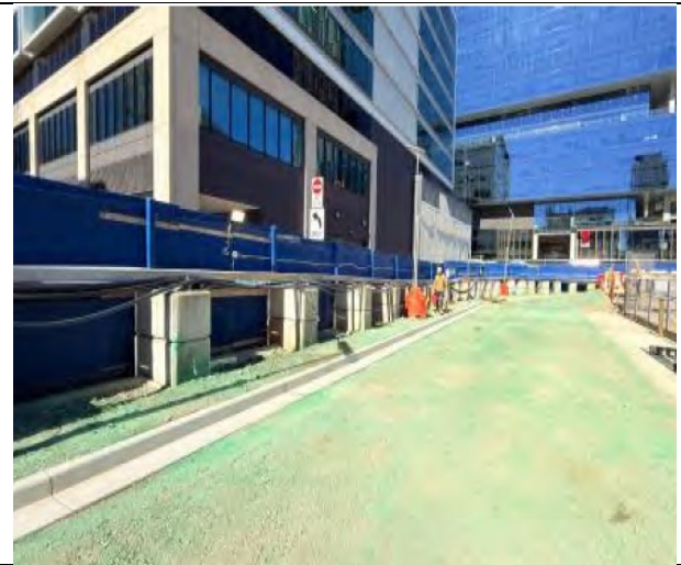
Figures 2.1 and 2.2 – Parramatta: Surface drainage works completed and polymer application observed (refer ER Inspection Section for action raised).
