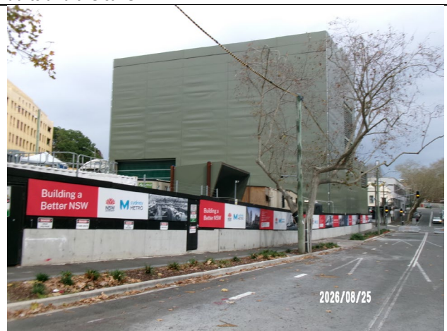
Figure 3.6 Pyrmont East: Viewed from Union Street.
