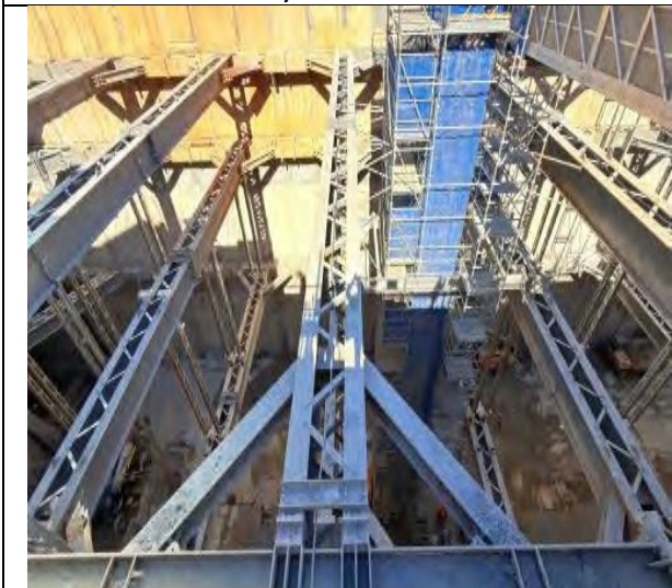
Figure 2.3 –Station Box, Parramatta: Hydro demolition of D-wall block outs continuing.
