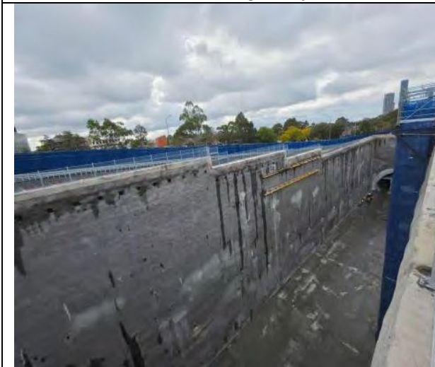
Figure 2.9 –Westmead: Hydro demolition of block outs in the station box. Power pack located on the surface (pad03).
