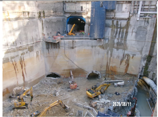
Figure 3.2 Hunter Street East: View of Bligh Street pedestrian adit and tunnels in eastern face of the excavation.
