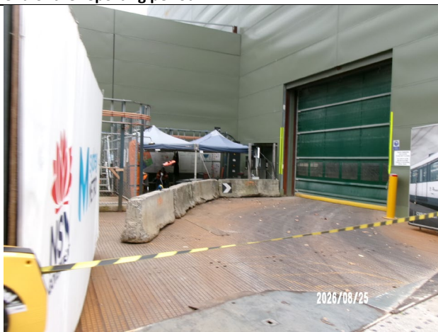
Figure 3.5 Pyrmont West: Acoustic shed access.
