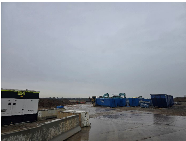
BRD – Civil works ceased and internal road conditions were managed during rainfall.
