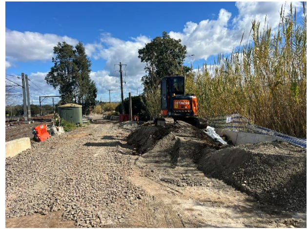
Laydown area 1: Stockpiles have been managed well with no offsite issues.
