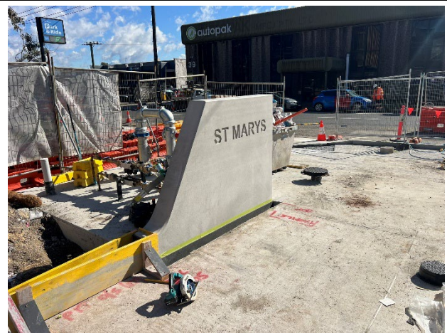
Harris Street / Compound: Signage is progressively being installed as per the PUDCLP.
