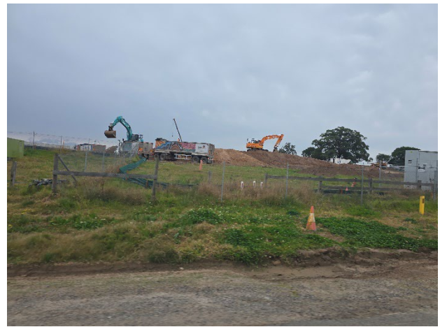
LUD/P1C – Precinct civil works commenced. ESC installed prior to earthworks commencing.
