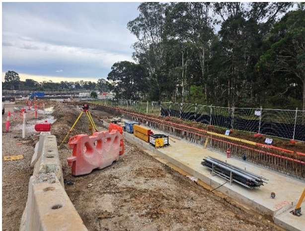
ORH - Retaining wall construction continued.
