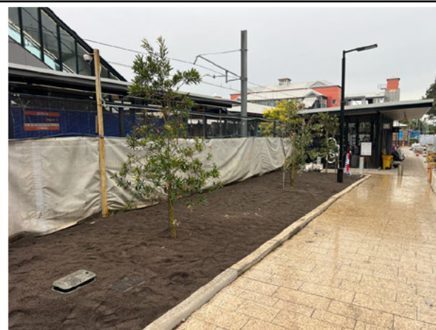
Northern Plaza: Landscaping has been successful; mulch will be the final surface treatment.
