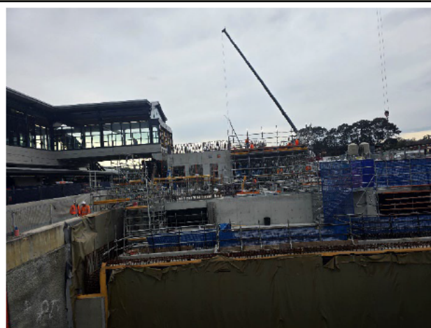
STM – Footbridge interchange to station.
