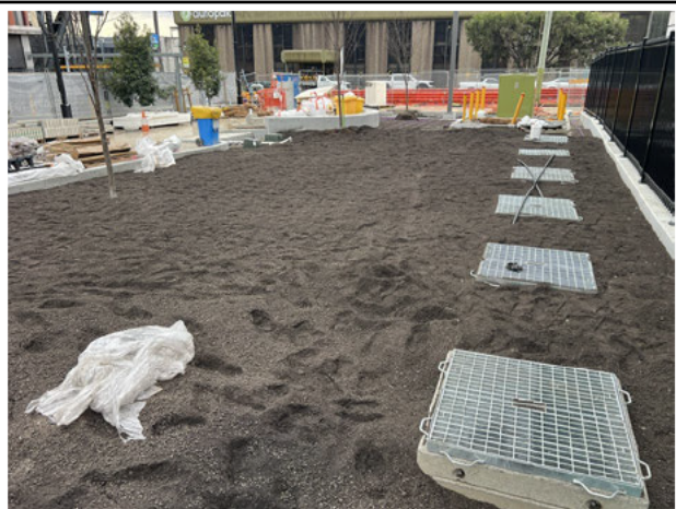
Compound: Landscaping commenced at the compound.
