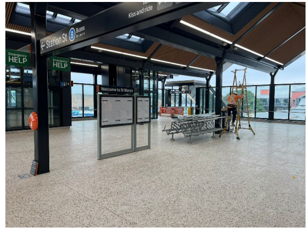
Overpass: Furniture and signs have been installed in the overpass.
