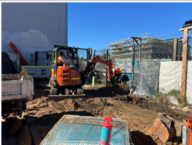
Compound: Excavation works were undertaken without issue.
