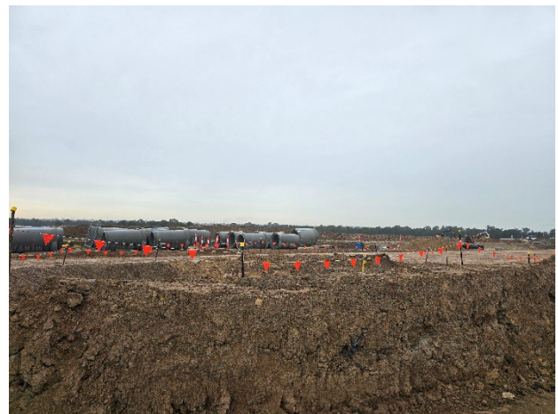
BRD – Innovation East stormwater installation continued.
