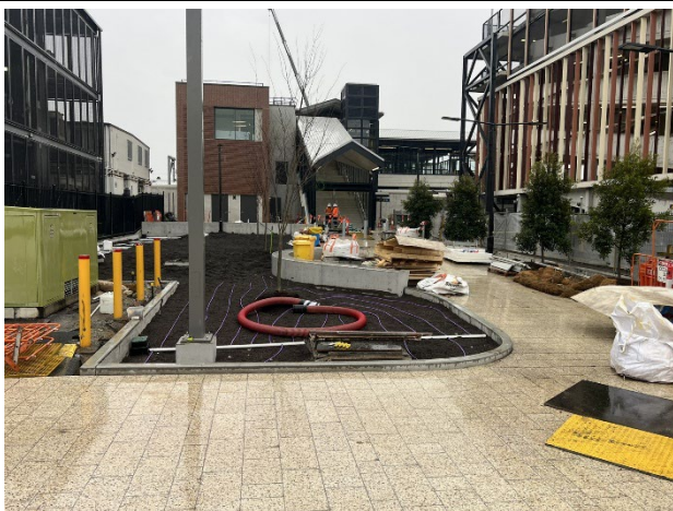
Harris Street: Paving on Harris St has now connected to the paved areas within the compound.
