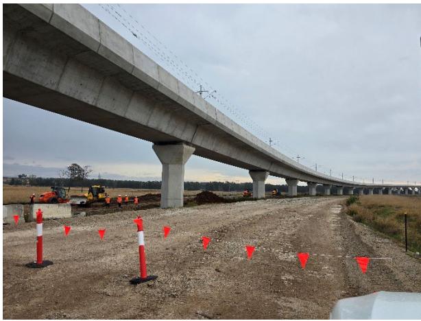
LUD - Permanent basin construction commenced.
