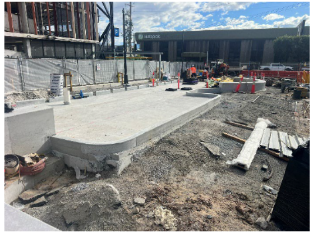
Compound: The concrete pours for the street furniture and walkway were undertaken without issue.
