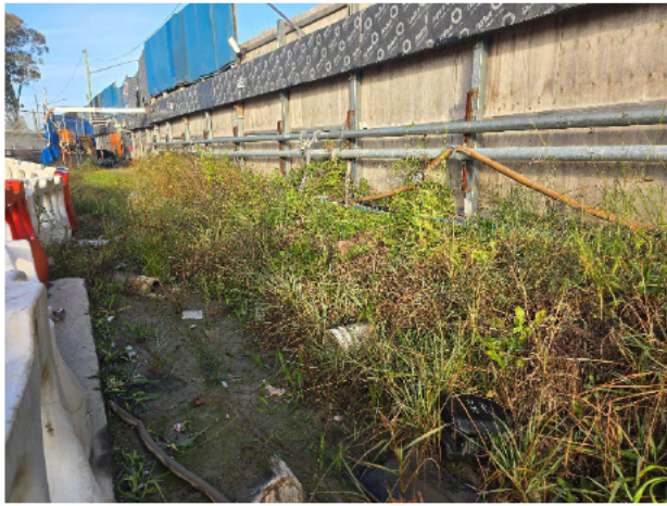
CMSF – Cleanup of the sump low point was required.
