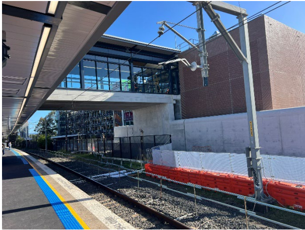
Platform 1/2: The overpass now has all of the glass installed.
