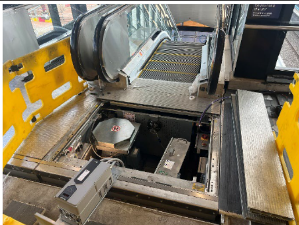
Overpass: Escalators are in the final installation phase with power being connected.
