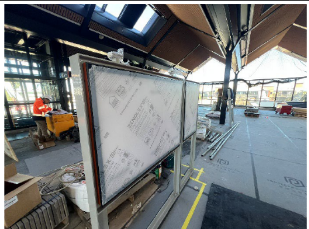
Overpass: Sign boards and furniture was progressively installed.
