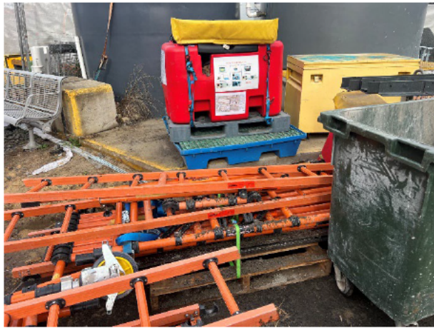
Compound: The fuel pod and spill kit were obscured by construction materials.
