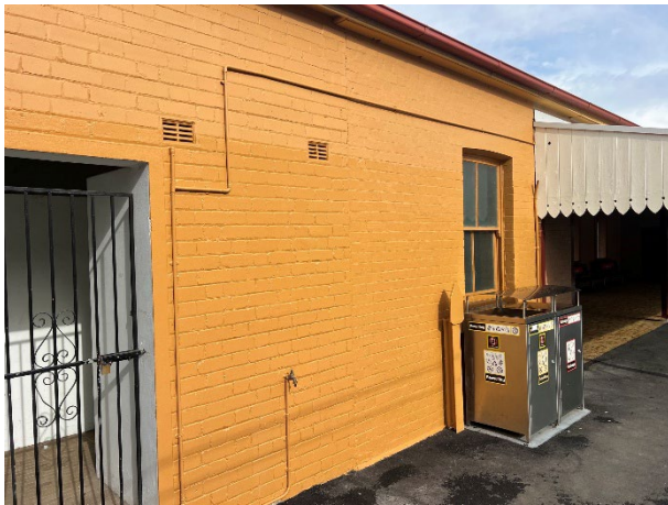
Platform 3/4: The station building has been painted its final colour.
