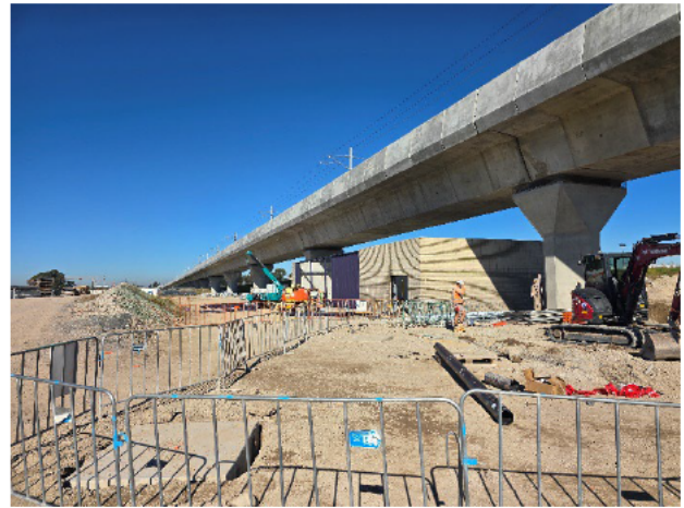
LUD – Water pipe defect repairs.
