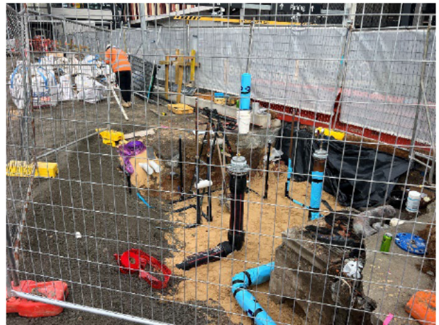
Compound: Fire main installation was completed adjacent to Harris Street.
