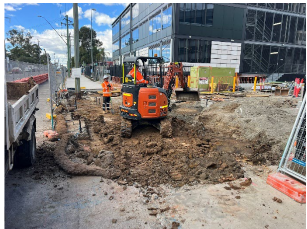
Harris Street: Works at the site compound driveway were occurring without issue, all material was cleaned up at the end of the shift.
