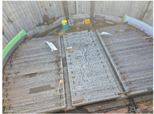
CMSF – Beam placement within the shaft was completed.
