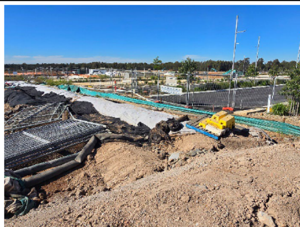
BRD – ESC was required for the basin discharge.
