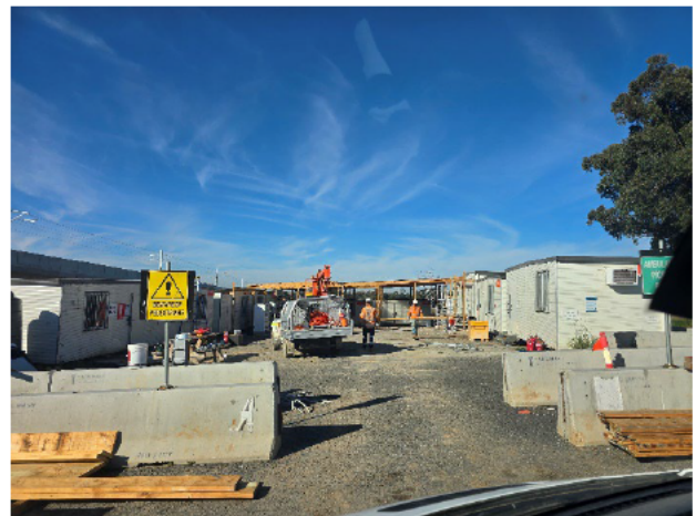
Luddenham to M12 – Site compound was being removed.
