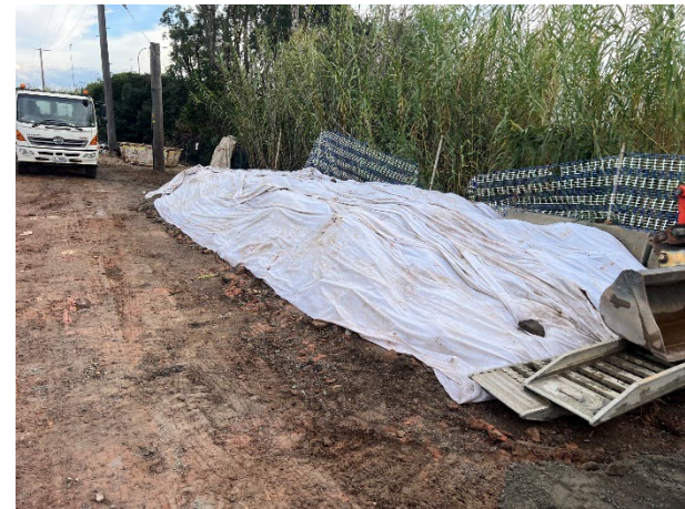
Laydown area 1: Stockpiles have been covered and contained within the stockpile boundaries.
