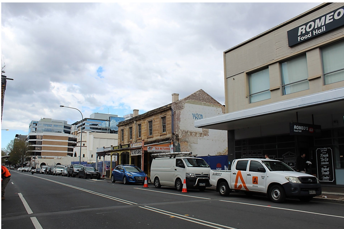
Figure 3.6: View looking southwest from the north side of George Street, after demolition works adjacent to the subject site. Source: OCP Architects, 5 September 2022.
