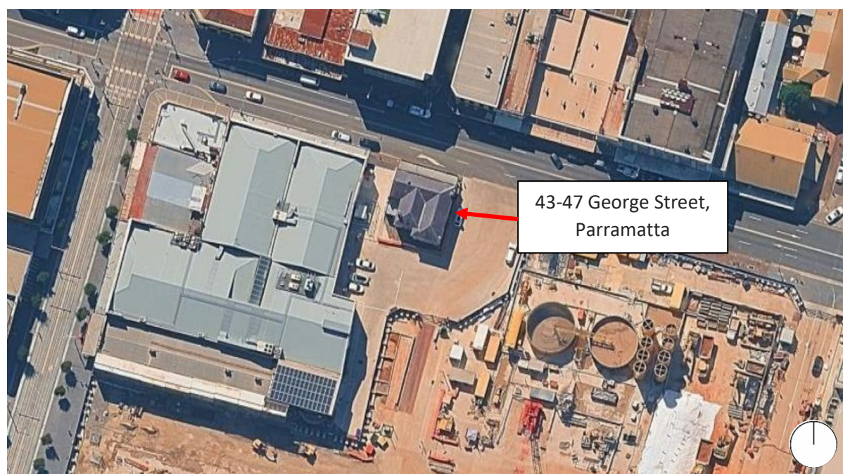
Figure 1.4: Aerial image showing the subject site at 43-47 George Street, Parramatta, following the extensive 2022-2023 demolition of neighbouring buildings. Source: Google Maps, accessed 15 April 2026.
