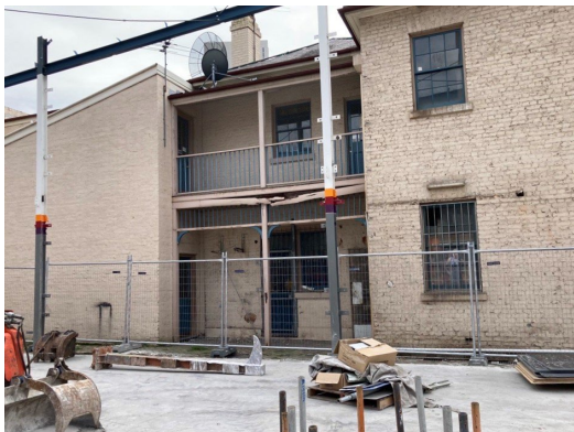
Figure 2.30: Rear elevation prior to demolition of two storey toilet wing (left) and rear balcony (centre). Source: Sydney Metro, June 2022.
