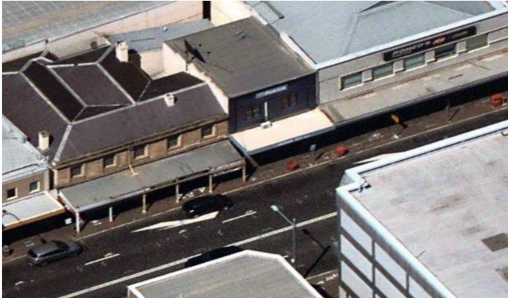
Figure 3.2: Oblique aerial image of the subject site from George Street in May 2022, prior to the demolition of the surrounding buildings. View looking southwest, showing the scale and form of the street with two storey buildings with awnings at ground floor level, and offices above on first floor level. Source: Nearmap, May 2022.
