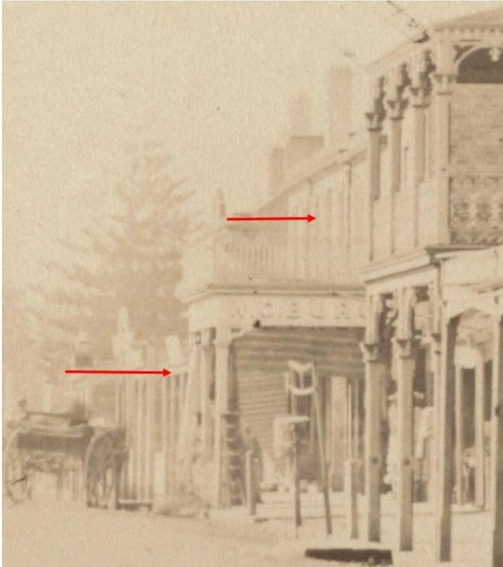
Figure 2.13: Excerpt of James Vickers' 1879 photograph of George Street, showing the George Street Shops - indicated by a red arrow - with the post-supported awning indicated by lower red arrow. Source: National Library of Australia.
