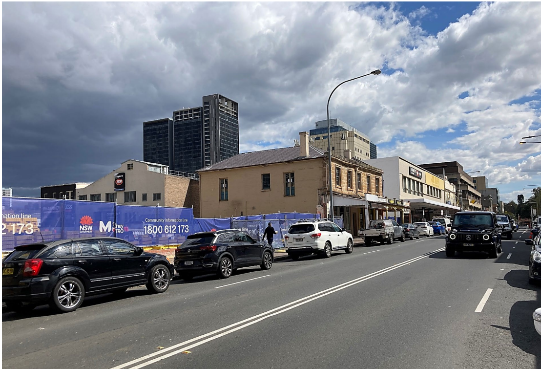
Figure 3.9: View south west towards the George Street Shops from the north side of George Street, after demolition works. Source: OCP Architects, 5 September 2022.
