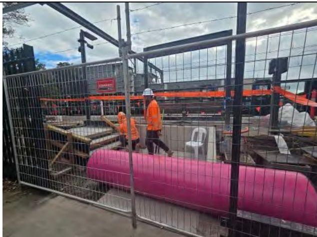
Figure 5 – Marrickville Station – Secondary egress works ongoing.
