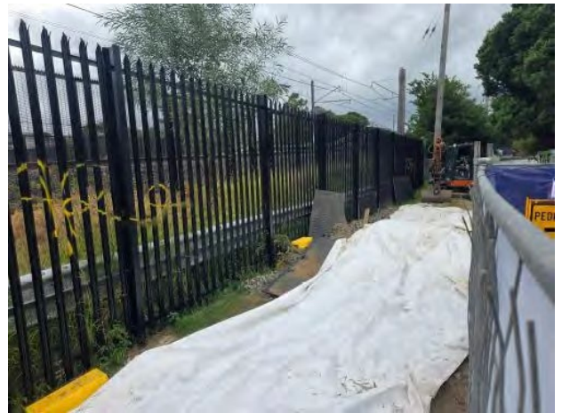
Figure 4 – Marrickville - Active Transport Link/Pedestrian and cyclist path works underway between Charlotte Ave and Riverdale Ave.
