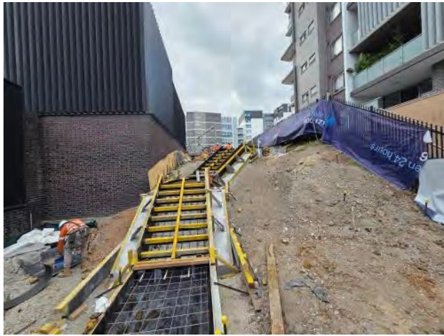
Figure 1 – Canterbury Station – Secondary egress works underway.
