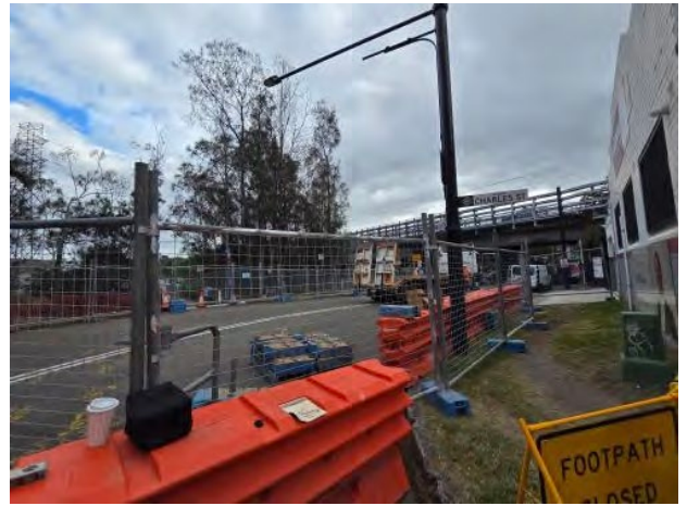
Figure 2 – Charles St – Overhead Crash Beam (OHCb) works underway. Traffic control and fencing installed. Erosion and sediment controls installed near bridge embankment.
