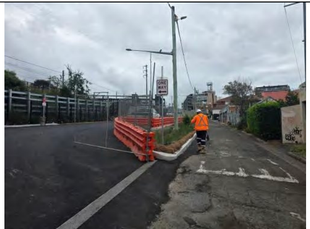
Figure 6 – Dulwich Hill Carpark - Landscaping works underway, asphaltting of carpark completed.
