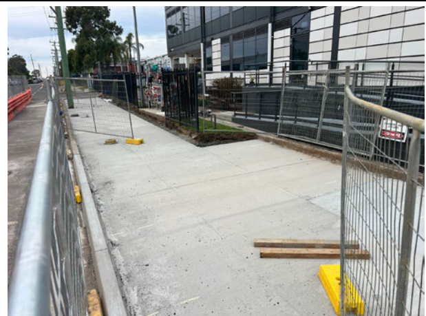
Harris Street: The footpath outside the site compound is progressing with paving due to be finalised in the coming weeks.
