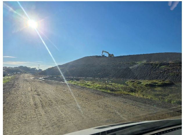
SMF – Reshaping of PS-102 continued.
