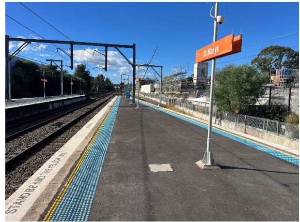
Platform 3/4: The tactiles and new platform pavement was installed.
