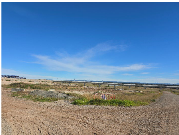
Water Pipeline to Luddenham Station –The stockpile area was generally maintained, and stockpile signage had been installed. Stockpile tracking registers continue to be updated.
