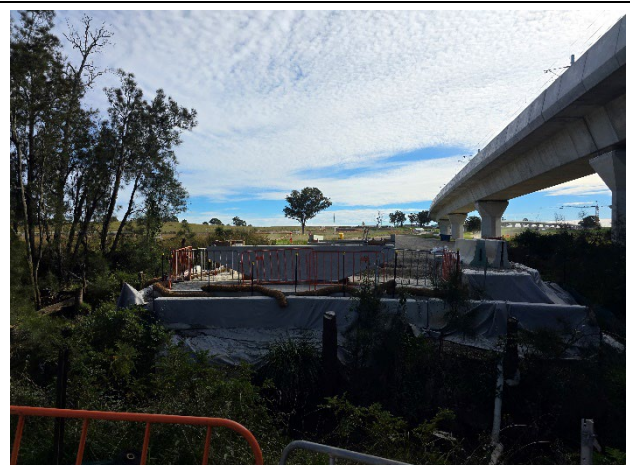
Luddenham to M12 – ATC Bridge 3 crossing was pending installation of precast slabs. Erosion and sediment controls were maintained.
