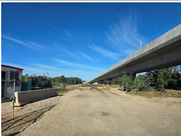
Patons Lane to water pipeline – Rumble grids were maintained and dust suppression was observed.
