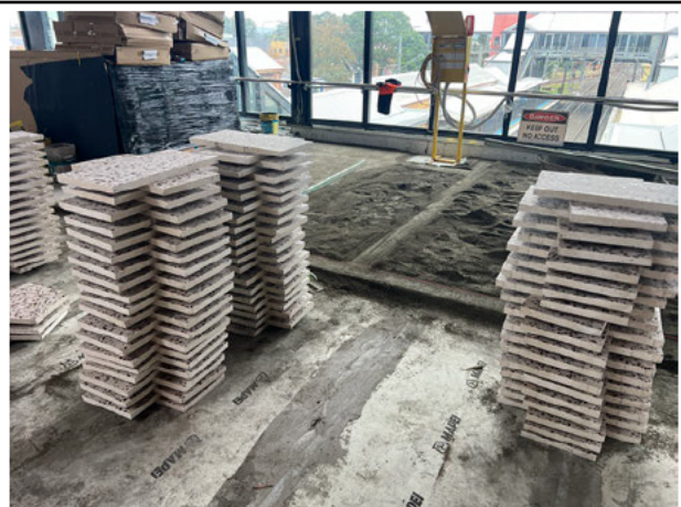
Overpass: Paving continued without issue in the overpass.
