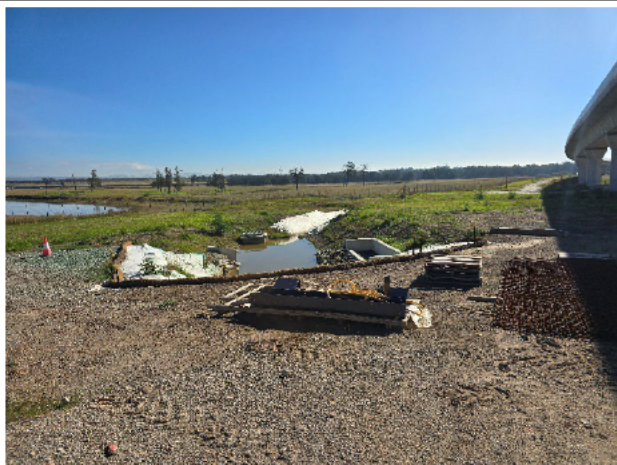
LUD – Sump erosion and sediment controls were in place.
