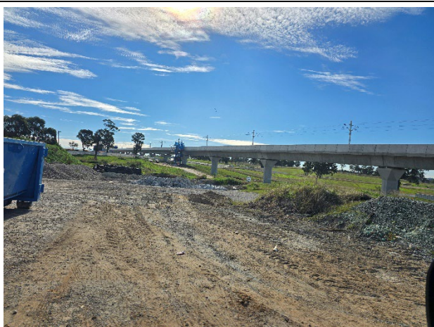
Luddenham to M12 – Concrete washout controls were maintained.
