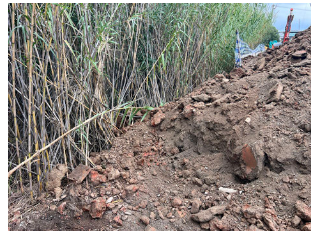
Laydown area 1: Unconsolidated material was stockpiled without adequate ERSSED controls and encroached on existing vegetation (weeds).
