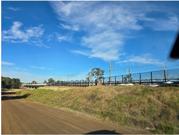
Lansdowne Rd to Patons Lane – Internal fence construction continued.
