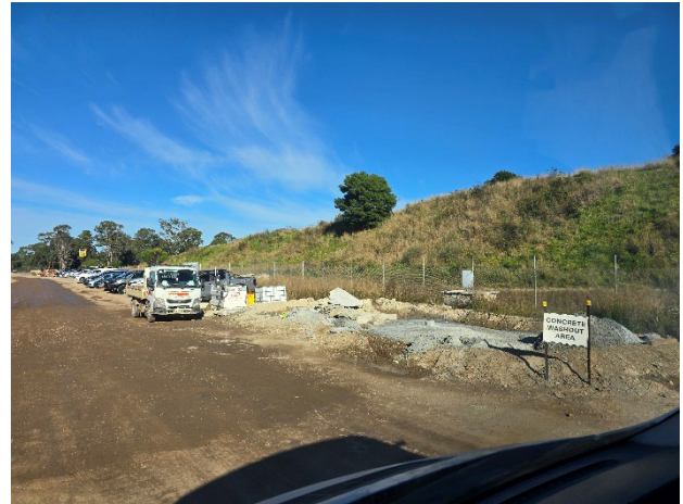
Lansdowne Rd to Patons Lane – Concrete washout controls were maintained.
