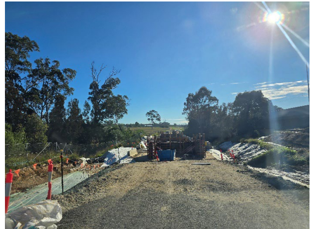
Lansdowne Rd to Patons Lane – Bridge 2 formwork was in place, with erosion and sediment controls maintained and polymer applied to batters.
