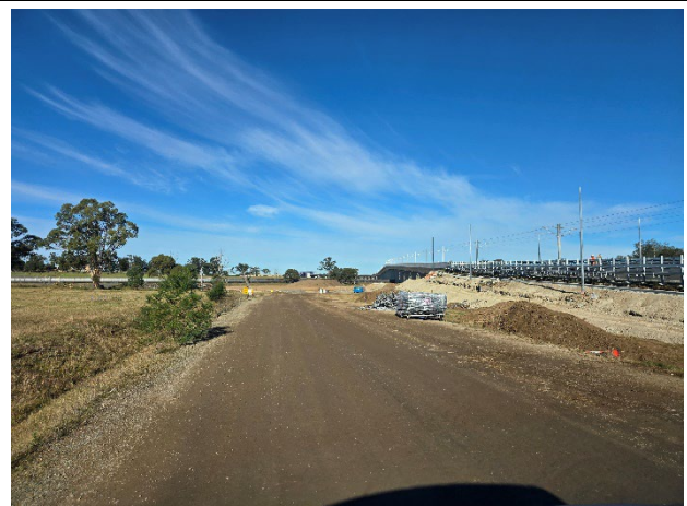
Patons Lane to water pipeline – Benching for internal fence installation continued, with clear polymer applied to batters.
