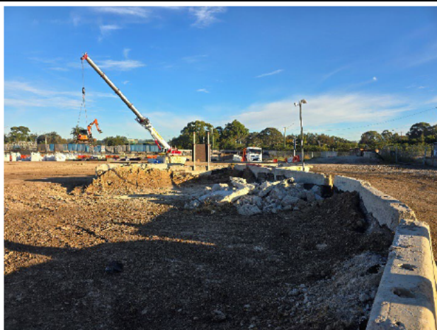
CMSF – Concrete washout area associated with STM works had been cleaned.
