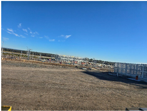
SMF – Train wash shed construction had commenced.
