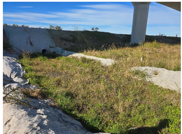
Water Pipeline to Luddenham Station – Clean water diversion was maintained adjacent to the emergency stairs.
