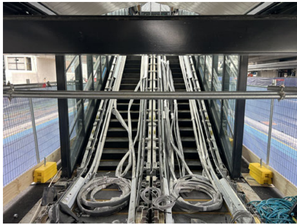
Platform 1/2: The escalators are being progressively installed on platform 1/2.
