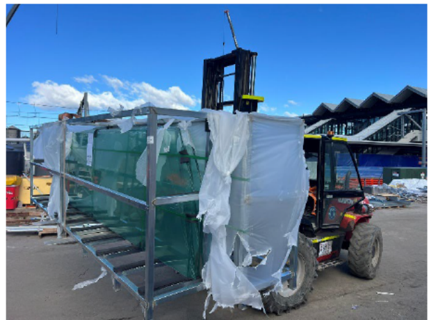
Compound: Glass panels were being unloaded for installation in the overpass.
