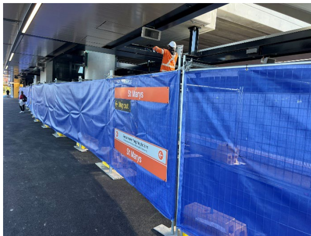
Platform 3/4: The plywood hoarding was removed as asphalt pavement now covers all disturbed areas.
