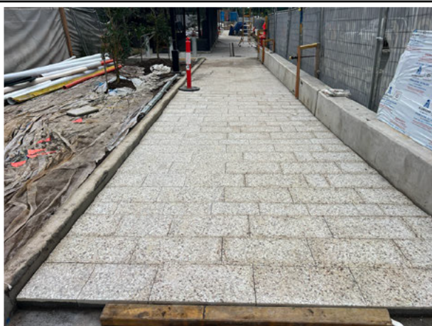
Commuter carpark: The paving progressed adjacent to the bike locker.
