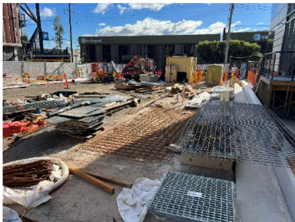
Compound: Aside from the rubbish bins, the compound was generally clean and tidy.
