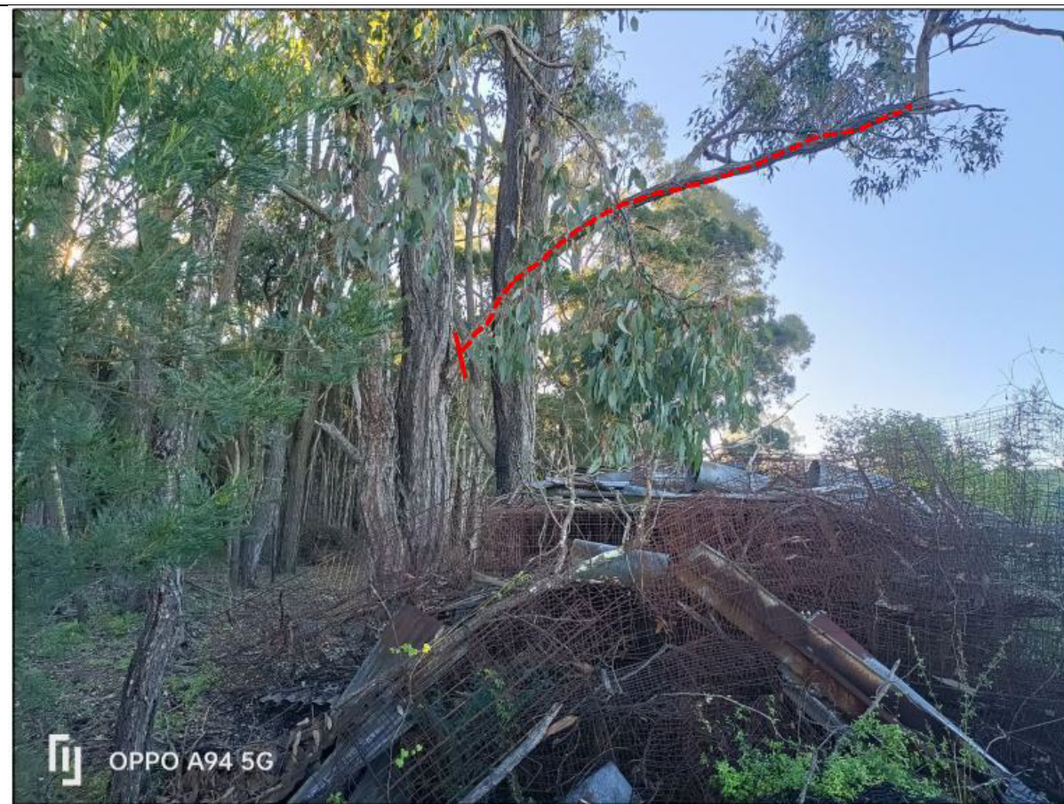
Figure 8 – Pruning required for retaining wall construction and rubbish removal
