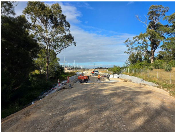
Lansdowne Rd to Patons Lane – ATC works at Blaxland Creek.
