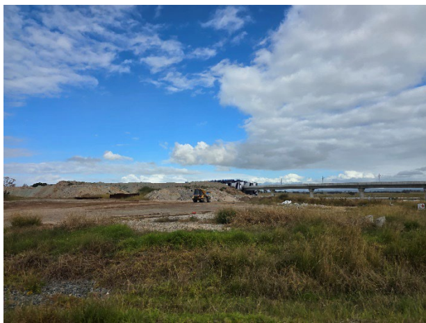
Water Pipeline to Luddenham Station – Stockpile area was generally maintained and stockpiles segregated. Stockpile tracking under investigation and signs were required.
