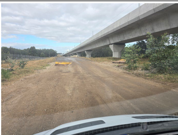
Patons Lane to water pipeline – Rumble grids were being maintained during the inspection on 12 May.
