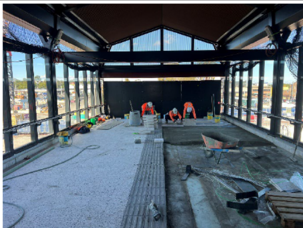
Overpass: Paving on the southern side of the overpass continues without issue.
