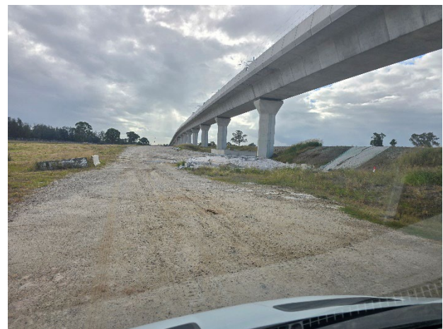
Water Pipeline to Luddenham Station – Management of runoff from recent concrete works was discussed with PLM, noting forecast rainfall, pooled water adjacent to the works, the sensitive receiver location and project discharge requirements.
