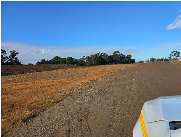
Lansdowne Rd to Patons Lane – Reshaping of area to the east of the alignment in preparation for topsoil placement.
