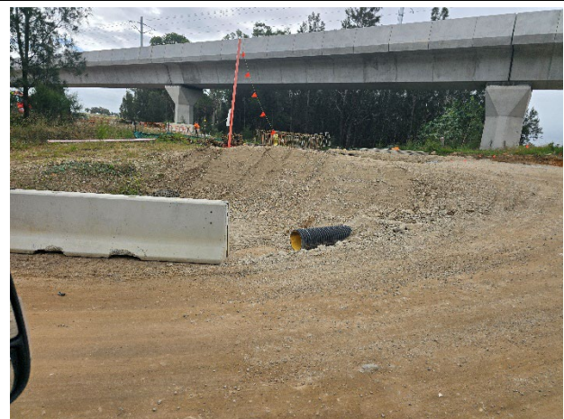
Luddenham to M12 – ESC was required for stormwater discharge pipe at the ATR creek crossing (PLM promptly closed the action).
