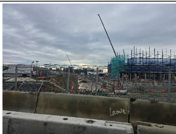
BRD – Western batter and southern station building.
