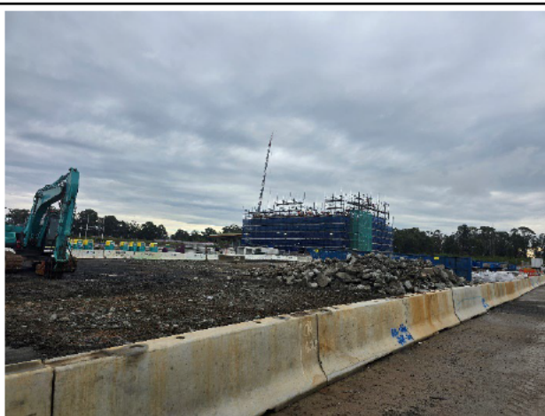
BRD – Concrete removal and northern station building.
