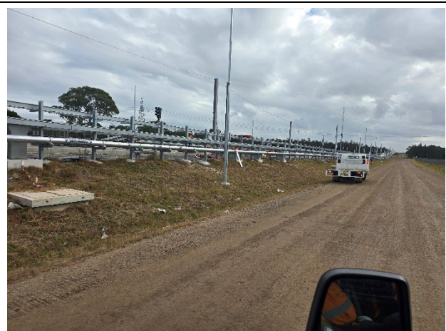
Patons Lane to water pipeline – Litter adjacent to Linewide workers 12 May.
