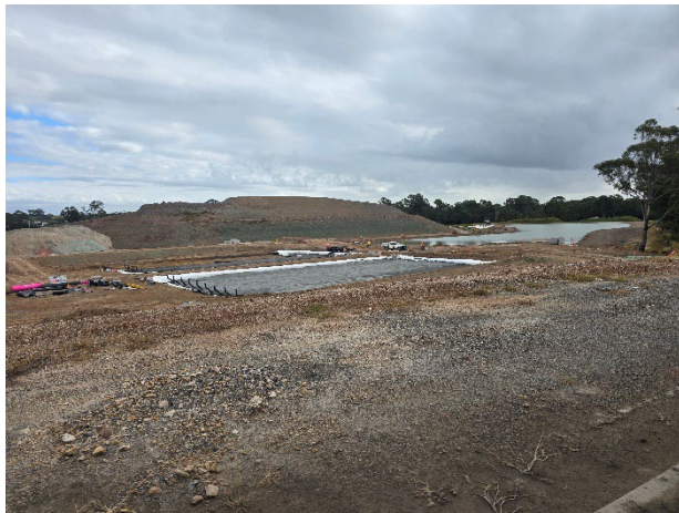
SMF – Lining for the permanent water basin.
