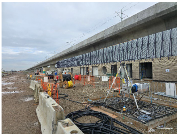
LUD – Station cladding works continued.
