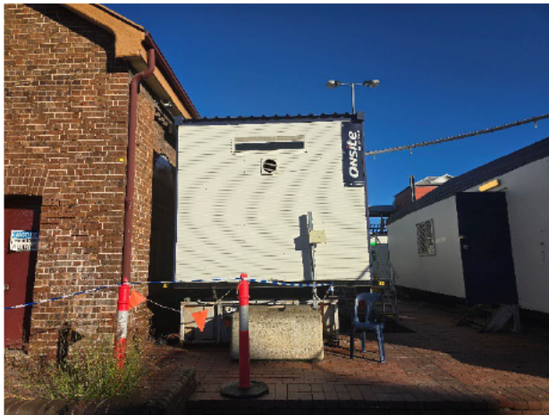
STM – portable sheds next to goods shed were removed.
