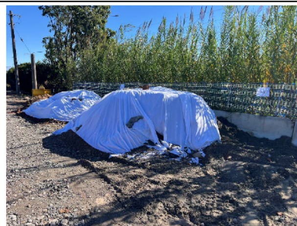
Laydown area 1: Covers were placed over stockpiled materials that aren't being used.
