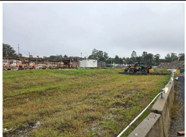
OHE – Demobilisation of Linewide sheds.
