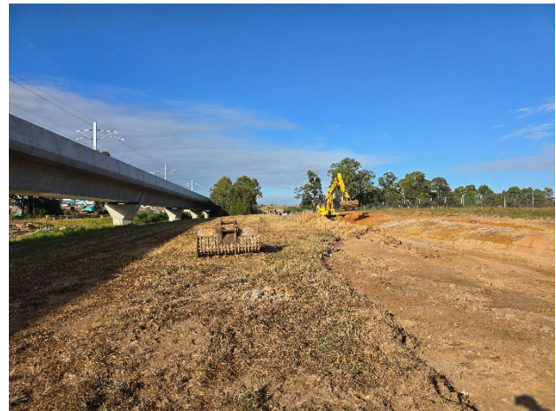
Lansdowne Rd to Patons Lane – ATC works north of Blaxland Creek.
