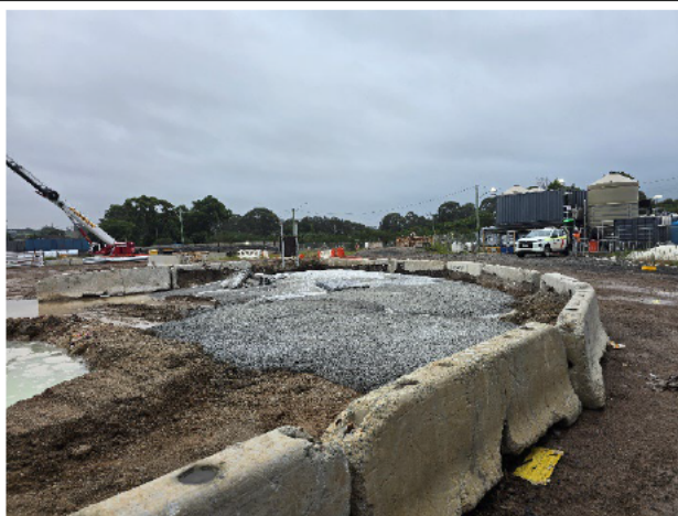
CMSF – Concrete washout from STM, noted captured in secondary bund.
