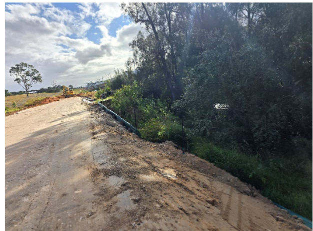
Lansdowne Rd to Patons Lane – Maintenance of ESC was required for ATC works at Blaxland Creek.
