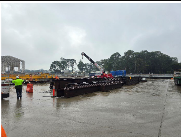
OHE – Removal of the gantry crane.
