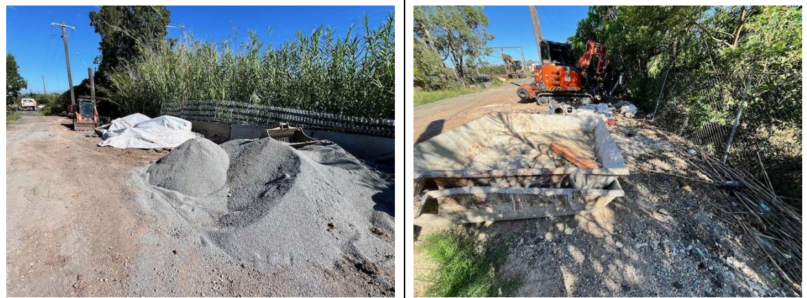
Photos 15-20: Material storage and stockpiling in Laydown 1. Location of concrete washout overflow incident.
