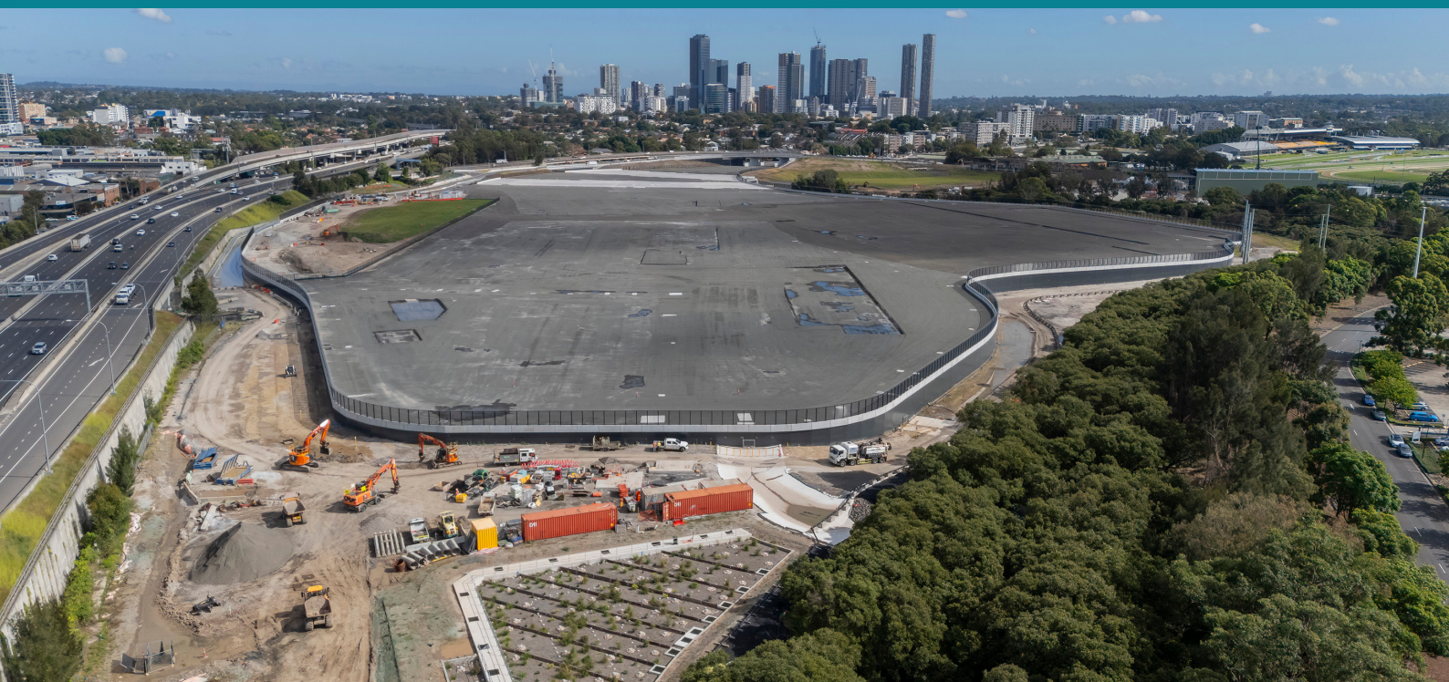
Clyde Stabling and Maintenance Facility site: preparing for the next stage.
