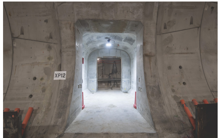
A completed concrete lined cross passage between The Bays and Pyrmont.
