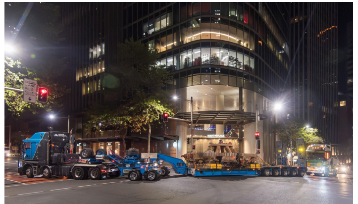
The complex removal of TBM Ruby's 90-tonne cutterhead at Hunter Street marked a significant achievement for the project.
