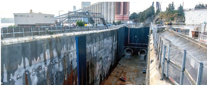
The Bays station box ready for linewise site establishment activities.
