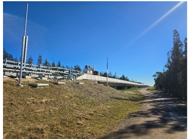
Patons Lane to water pipeline – Cable pulling works.
