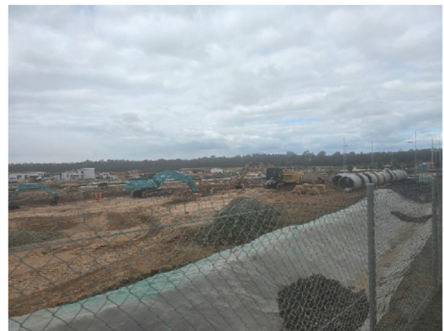
BRD – Stormwater pipe installation Innovation East.
