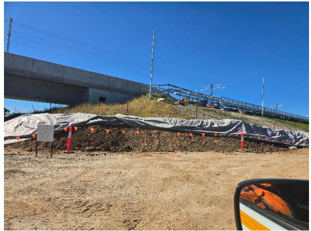
Luddenham to M12 – Stockpile required Geofab to be reinstated and pinned.
