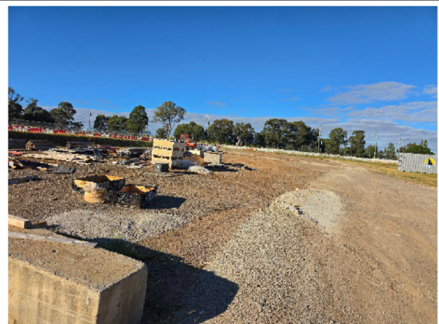
CMSF – Cleanup of laydown areas had occurred.
