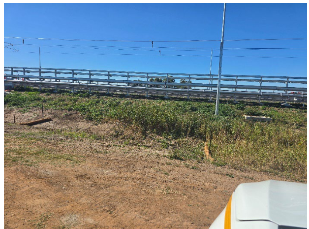
M12 to Elizabeth Dr – Coir logs were installed in drainage swales.
