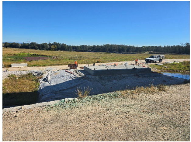
Water Pipeline to Luddenham Station – Pad for emergency egress stair construction.
