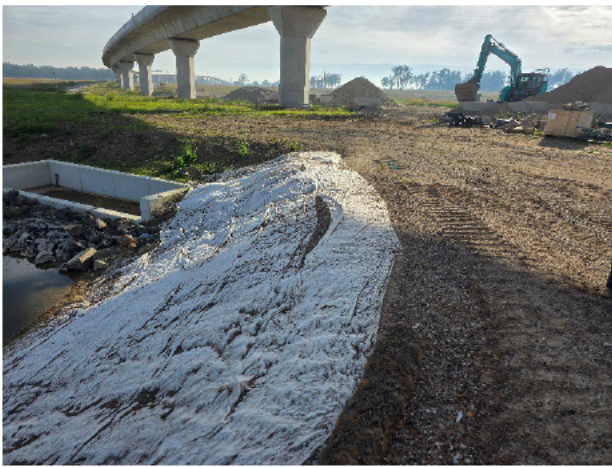
LUD – Temporary sump required inlet protection (closed during the inspection).
