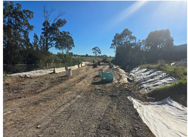
Lansdowne Rd to Patons Lane – Piling work completed, breakback to commence.
