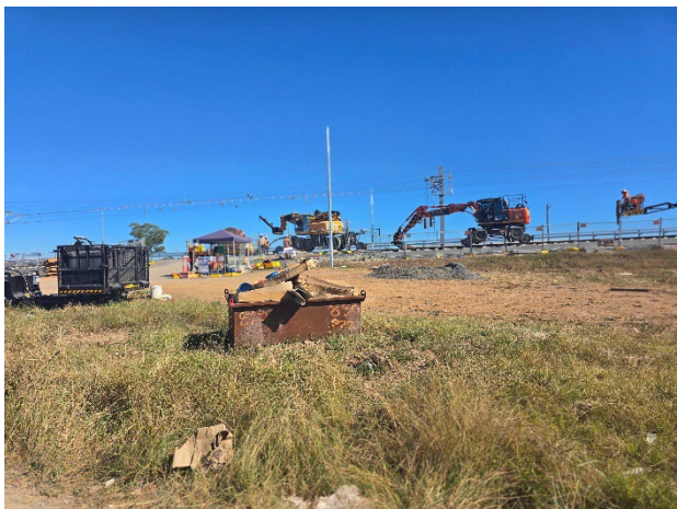
M12 to Elizabeth Dr – Cable pulling continued.
