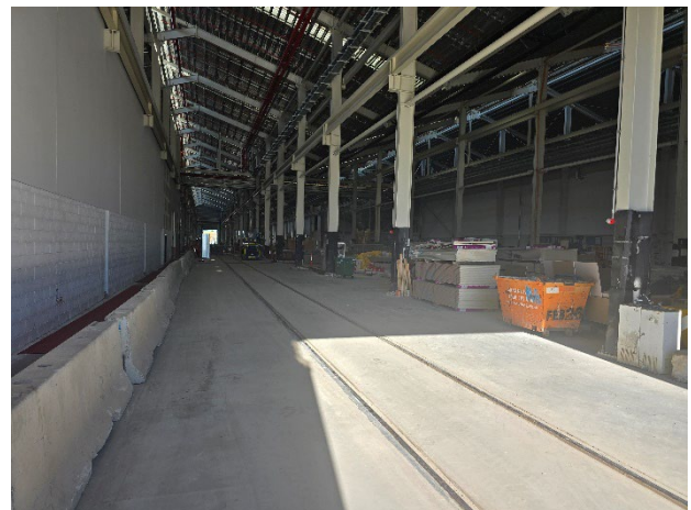
SMF – Maintenance facility was tidy.
