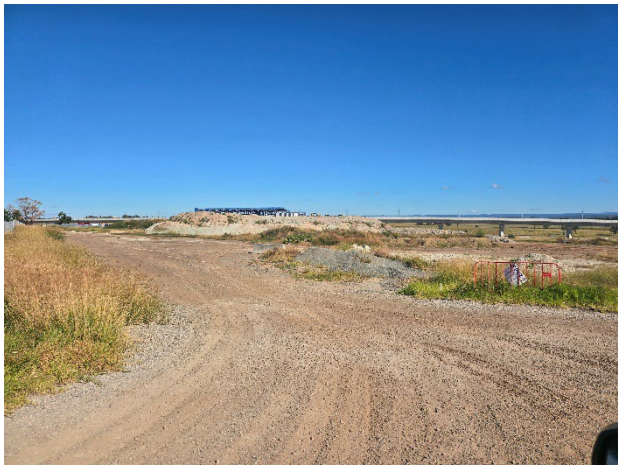
Water Pipeline to Luddenham Station –Stockpile area was generally maintained and stockpiles segregated.
