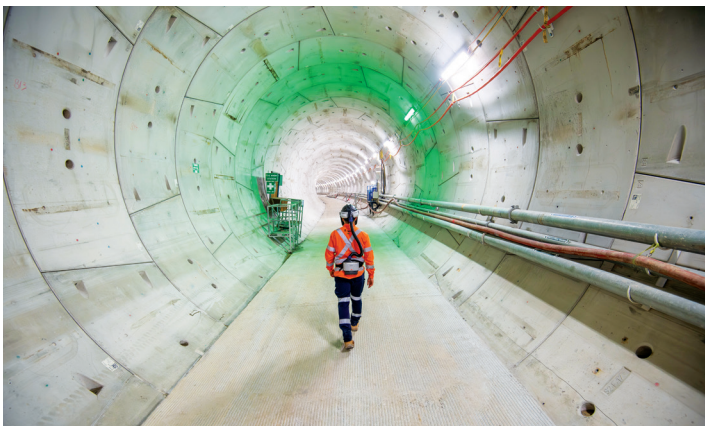
Inside the metro tunnels between Pyrmont Station and Hunter Street Station.
