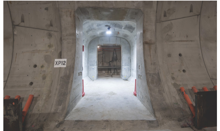
A completed concrete lined cross passage between The Bays and Pyrmont.
