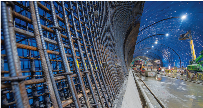
Steel reinforcement is installed prior to the permanent concrete lining.
