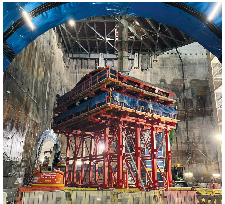
Part one of three formwork pieces in Pymont West.
