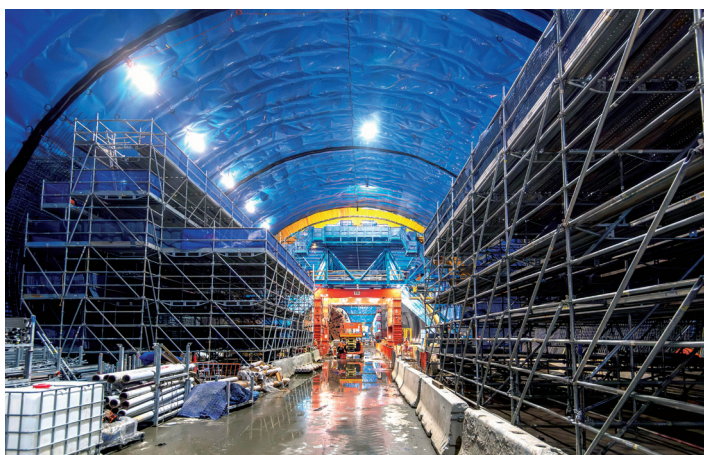
Permanent concrete lining works continue in the station cavern.
