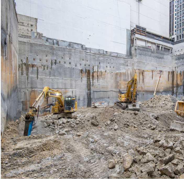
Excavation in the Hunter Street West shaft.
