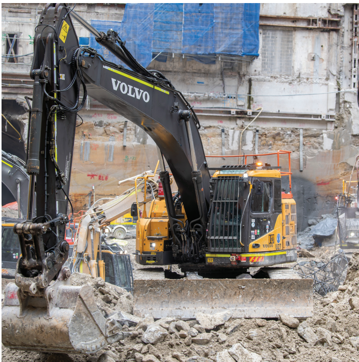
Excavation of the second stage of Hunter Street East is underway.
