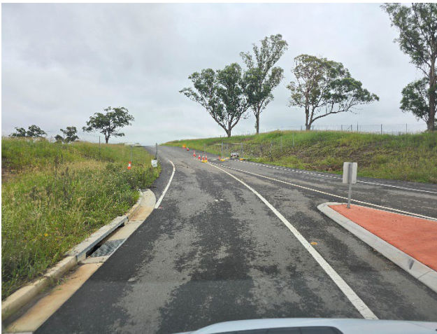
Water Pipeline to Luddenham Station – Site access was maintained.
