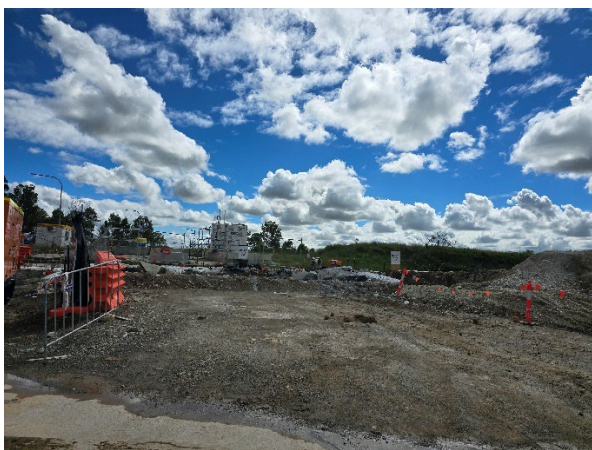
BRD – Concrete washout area was maintained.
