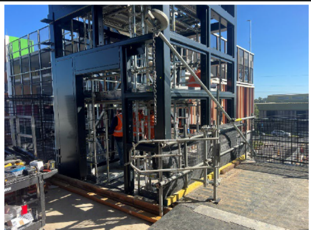
Overpass: Lift works have commenced with minimal environmental risk.
