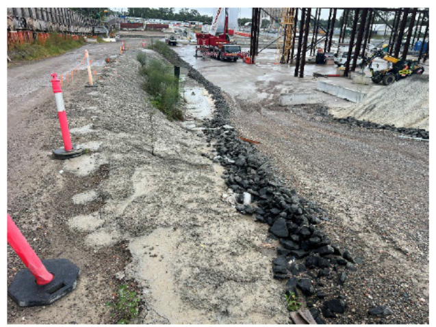
OHE – Kent Rd widening work batter required litter removal.
