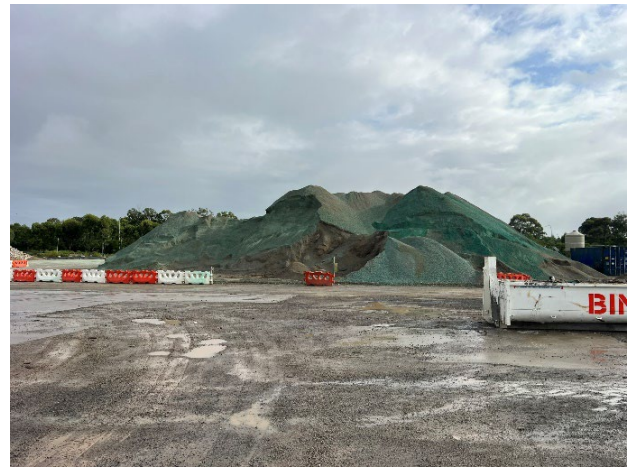
OHE – Polymer had been applied to the crushed concrete stockpile.
