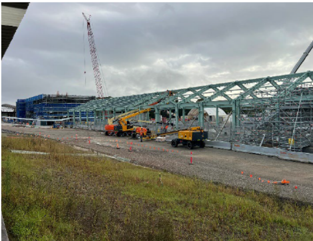
OHE – Construction of the station aboveground buildings.
