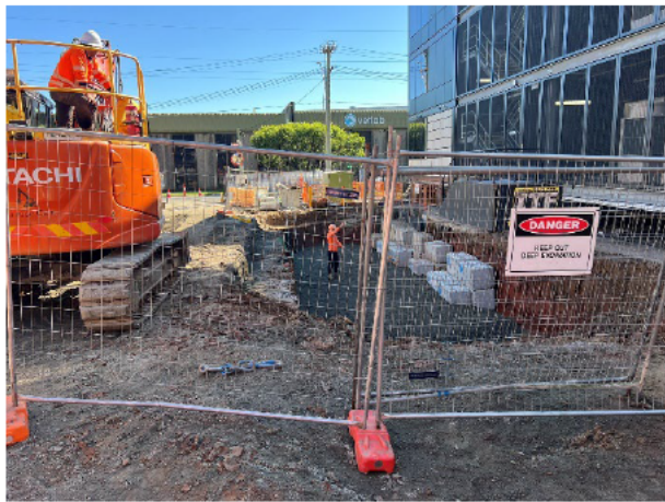
Compound: Service works are ongoing in the compound.
