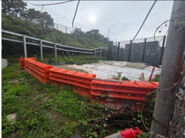
Figure 3 – Ness Street, Dulwich Hill – Planning underway for pedestrian/cyclist bridge piling works.
