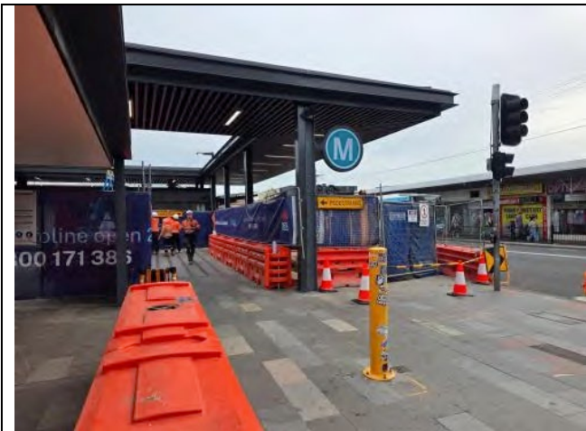
Figure 5 – Campsie Station – Utility relocation works commenced.
