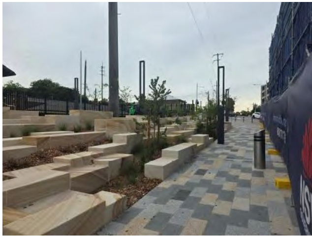
Figure 1 – Dulwich Hill Plaza works completed, area opened to the public.
