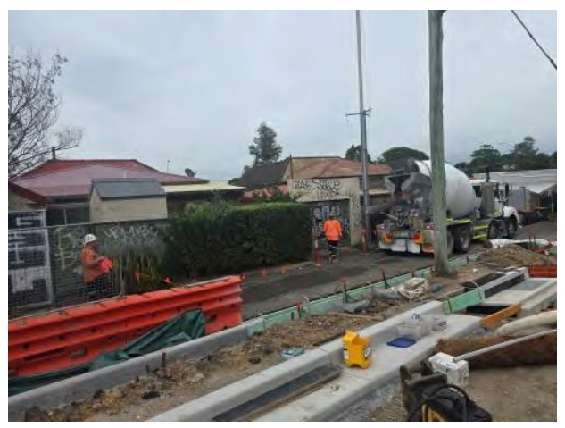
Figure 2 – Dulwich Hill – Kerb and gutter, landscaping and pavement works ongoing.
