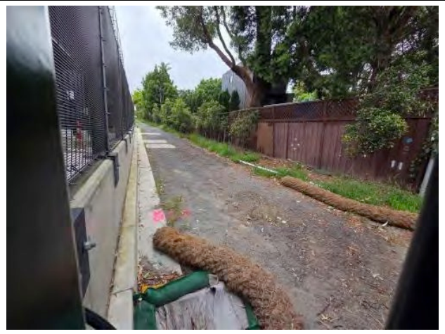
Figure 4 – Hurlstone Park MSB – Environmental controls in place around the stormwater drains.
