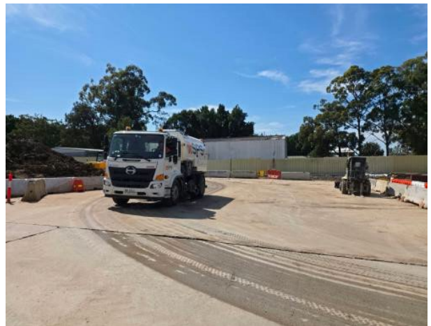
Figure 2.10 – Clyde Dive: Observed wet down of hardstand areas.
