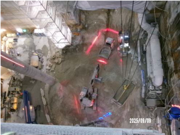
Figure 3.7 Pymont West: Load out of spoil ongoing.
