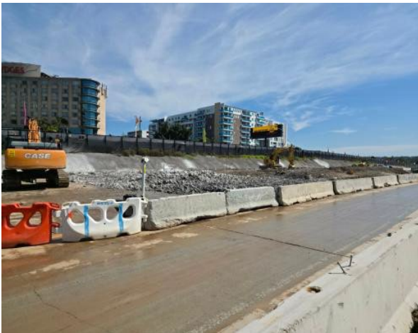
Figure 2.11 – Clyde Dive: Removal of concrete hardstand areas.
