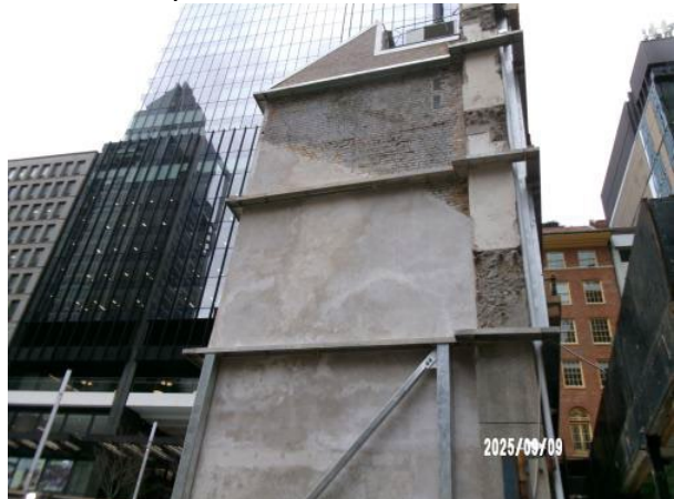
Figure 3.4 Hunter Street West: Strengthening works at Skinner's Hotel nearing completion.
