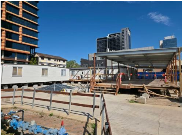
Figure 2.5 – Parramatta Site: Dismantling of previous site office sheds and amenities.
