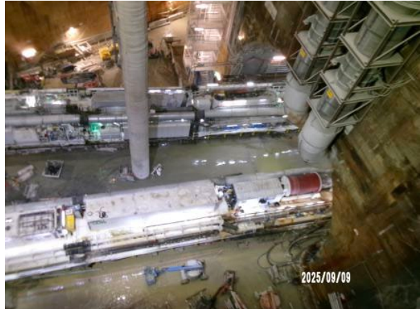
Figure 3.6 Pyrmont East: Both TBMs traversed through the caverns.
