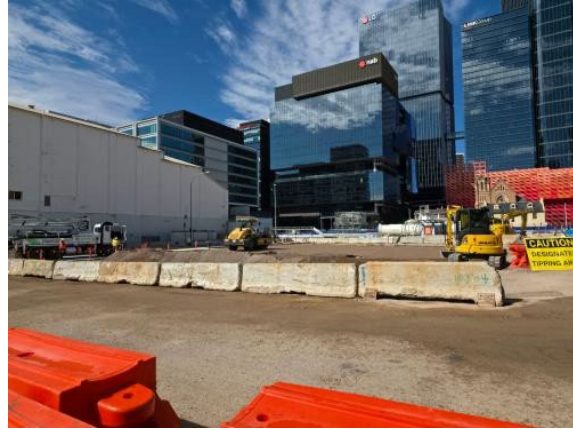
Figure 2.2 - Parramatta Site: Backfilling and compaction works.
