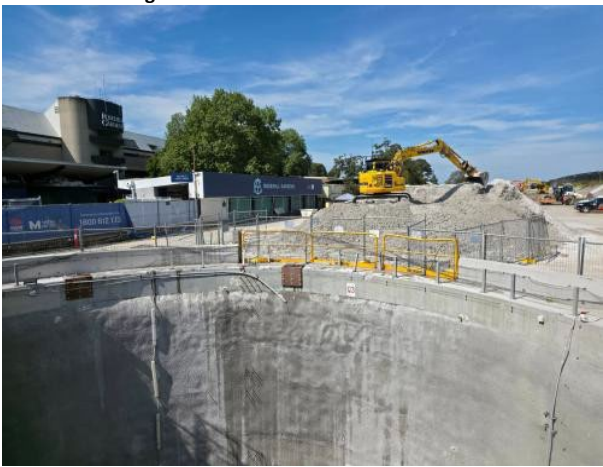
Figure 2.9 – Clyde Dive: Shaft backfilling works.
