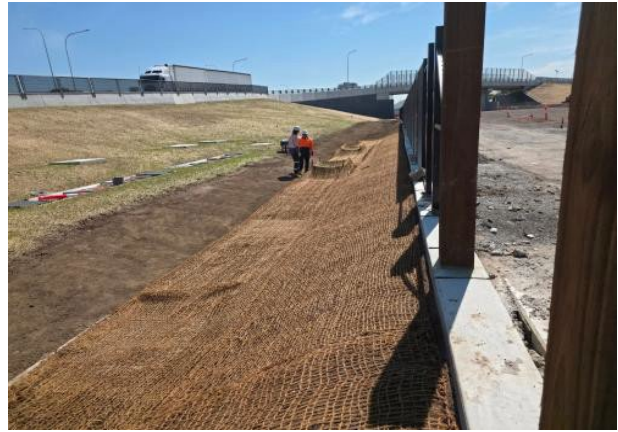
Figure 2.8 – Clyde MSF: Security fence and jute mesh installation works.
