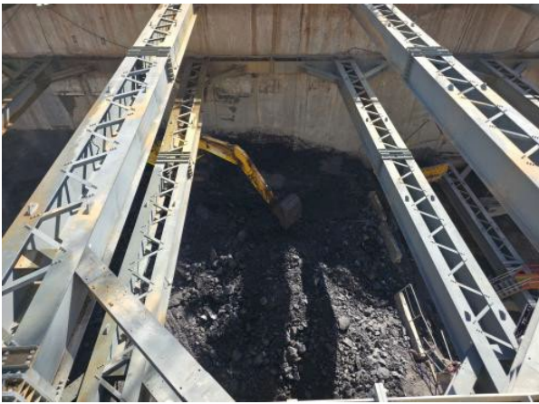
Figure 2.3 – Parramatta Site: Western Station Box – excavation works underway.
