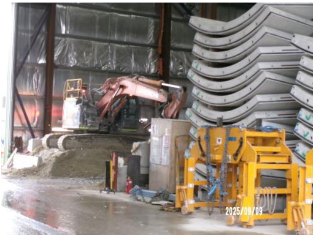
Figure 3.9 The Bays: A spoil stockpile area has been set up under the segment shed to receive and handle spoil loadout to the shed.
