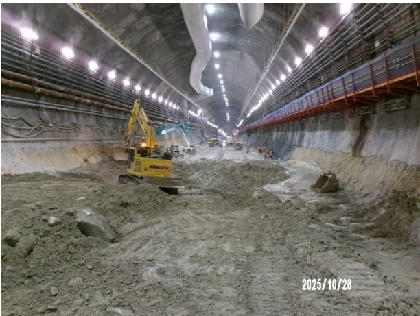
Figure 3.5 Pyrmont East: Near completion of the excavation of the station cavern.
