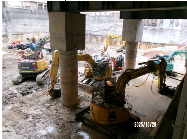
Figure 3.4 Hunter Street West: Ongoing bulk excavation of the shaft.
