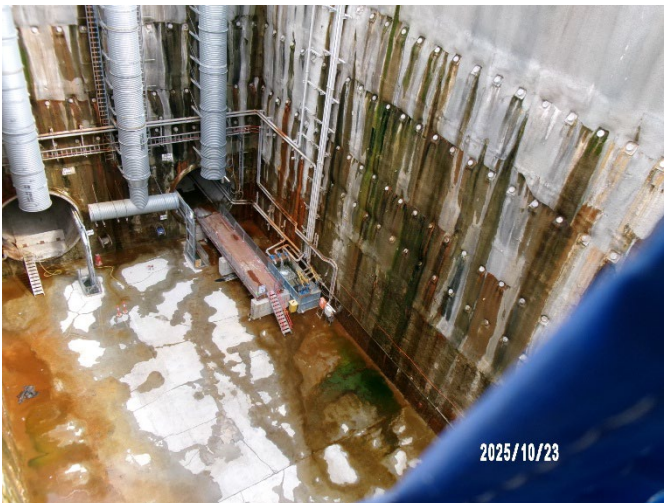
Figure 1.1 Station Box (The Bays) - Minor tunnel rectification activities ongoing.
