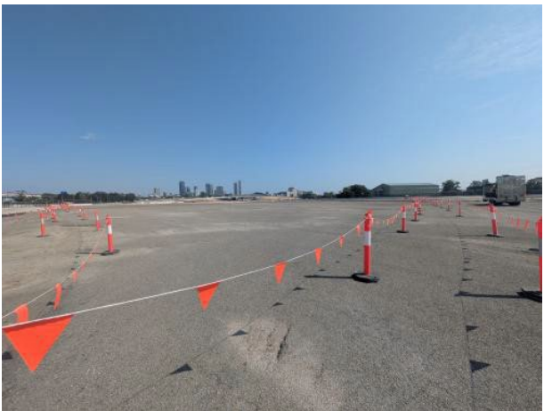
Figure 2.11 – Clyde MSF: Spray seal application.
