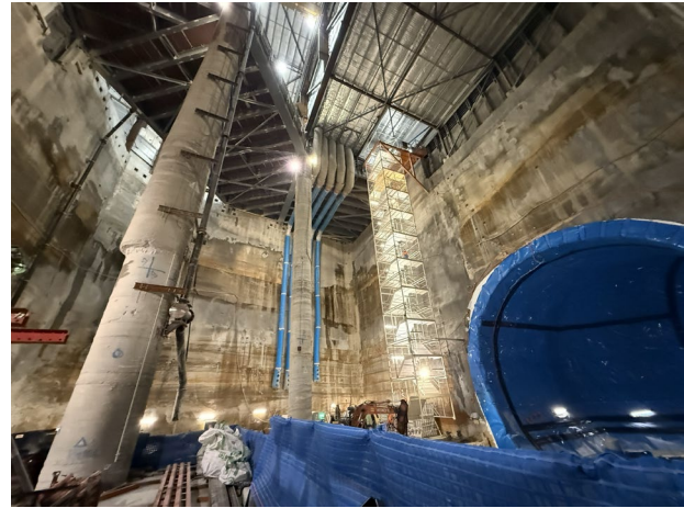
Figure 3.8 Pyrmont West: View from base of the shaft.
