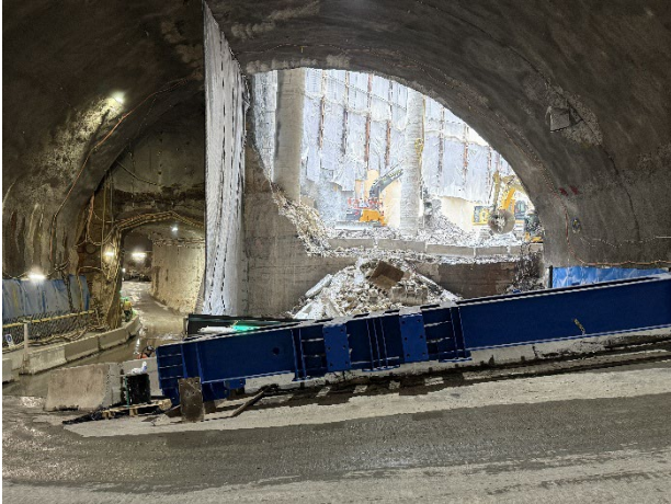
Figure 3.1 Hunter Street East: View from cavern into base of shaft excavation.
