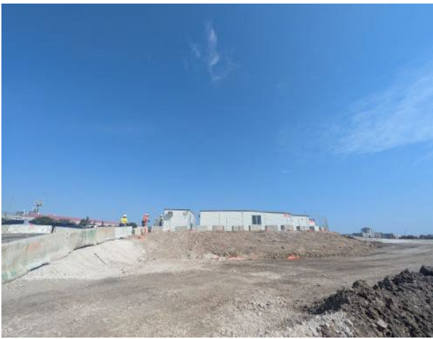
Figure 2.9 – Clyde MSF: MSF Crib shed repositioning continuing.
