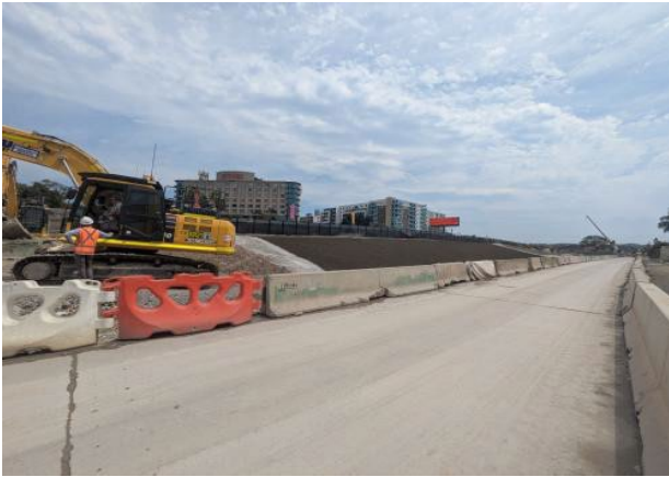
Figure 2.7 – Clyde Dive: Section of embankment spray sealed.
