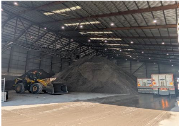
Figure 2.14 – Rosehill: Spoil storage and loading operations within shed.
