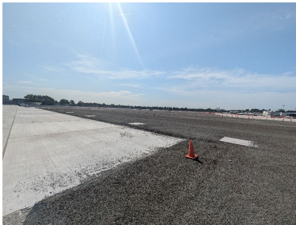
Figure 2.12 – Clyde MSF: Spray seal application.
