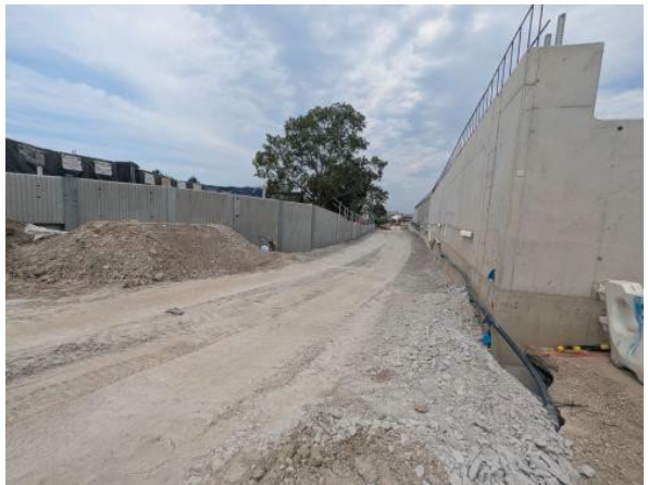
Figure 2.6 – Clyde Dive: Concrete hardstand removal and haul road fill placement.
