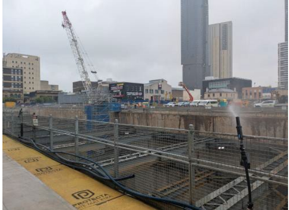
Figure 2.2 - Parramatta Site: Mistlers in operation for dust suppression.
