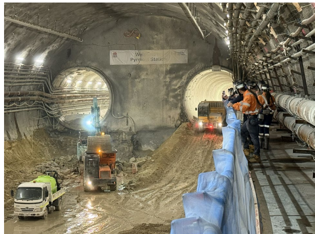
Figure 3.6 Pyrmont West: TBM tunnels from cross over cavern.
