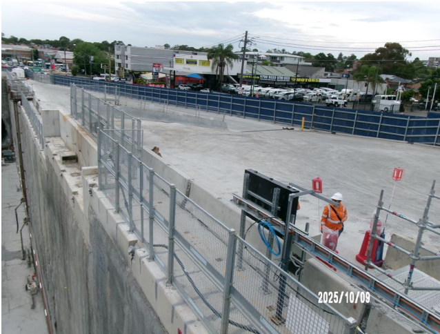
Figure 1.5 Site locked up and no workforce at the surface (Burwood North).
