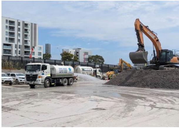
Figure 2.8 – Clyde Dive: Water cart mobilised.
