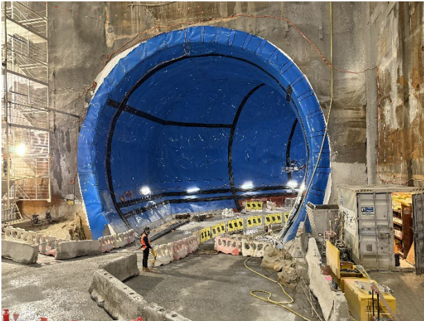
Figure 3.7 Pyrmont West: Service adit water proofing completed.
