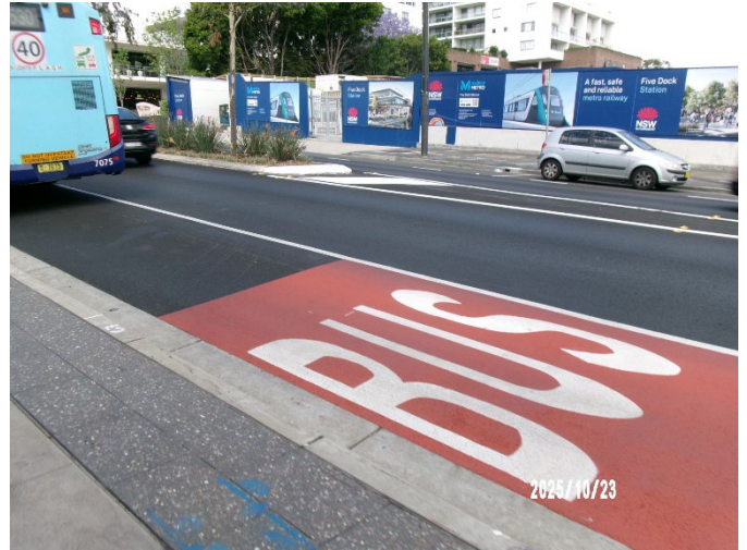
Figure 1.4 Western Shaft – recent resurfacing of the Great Northern Road has been completed by others (not AFJV) (Five Dock).
