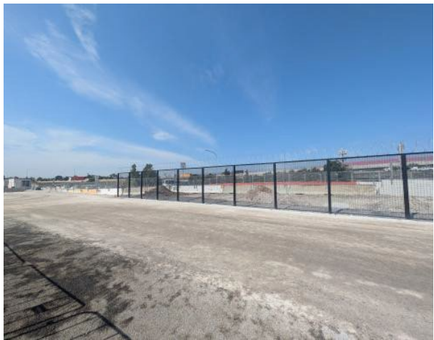
Figure 2.10 – Clyde MSF: Fence installation works continuing.
