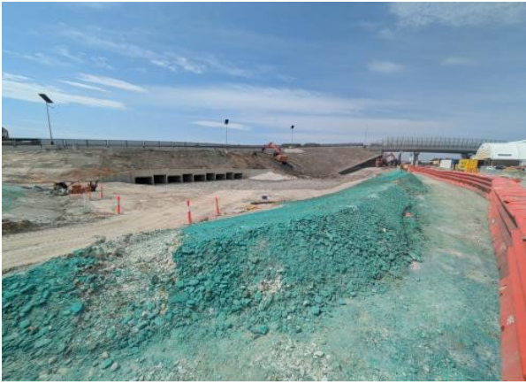
Figure 2.13– Clyde MSF: Preparatory works on embankment for landscaping.
