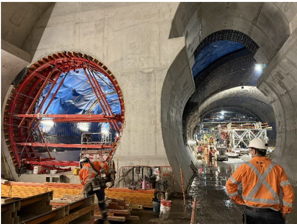
Figure 3.3 Hunter St East: Concrete works in turn back caverns.
