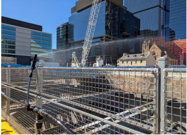
Figure 2.2 - Parramatta Station Box: Misters in operation (surface level) for dust suppression.
