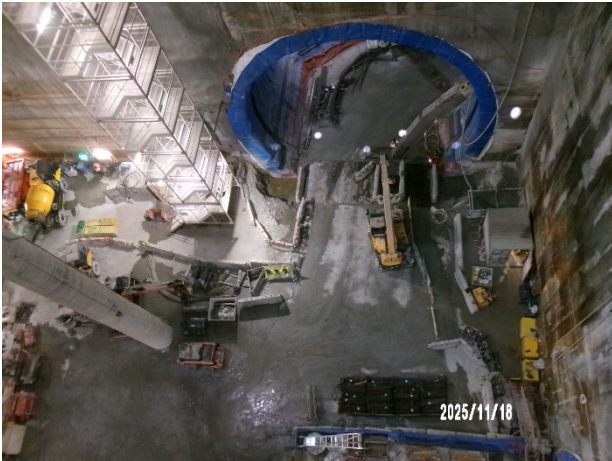
Figure 3.7 Pyrmont West: Service adit works.
