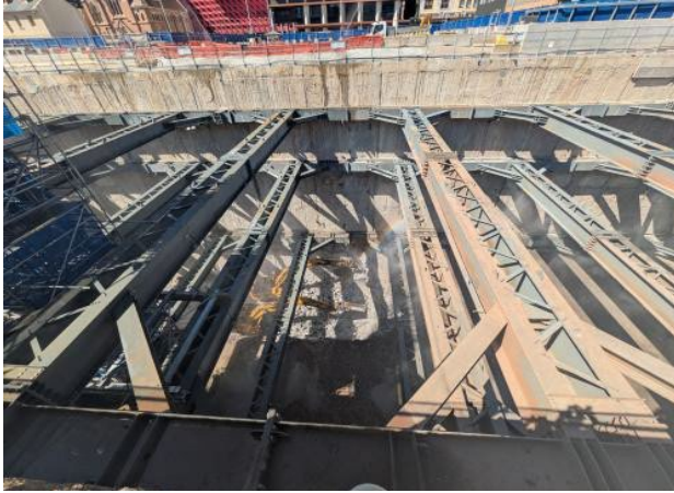
Figure 2.1- Parramatta Station Box: Hammering within box, with misters for dust suppression operational within the box.
