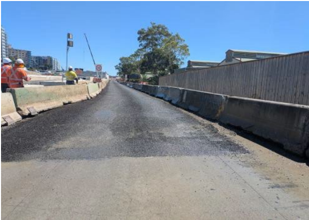
Figure 2.13– Clyde Dive: Chip seal applied on haul road (eastern boundary).
