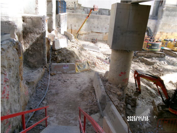
Figure 3.3 Hunter St West: Ongoing excavation of the shaft.
