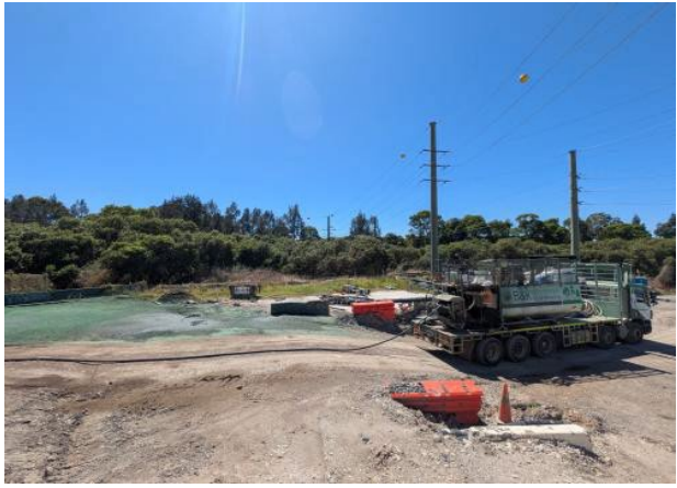
Figure 2.8 – Clyde MSF (West) - Hydro mulch application near retaining wall.
