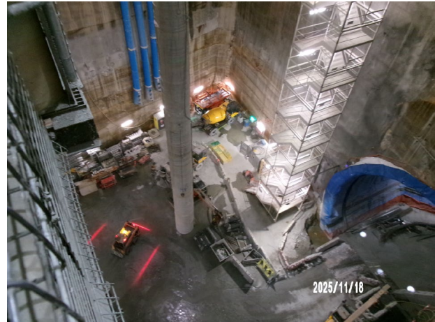
Figure 3.8 Pyrmont West: Base of west shaft.
