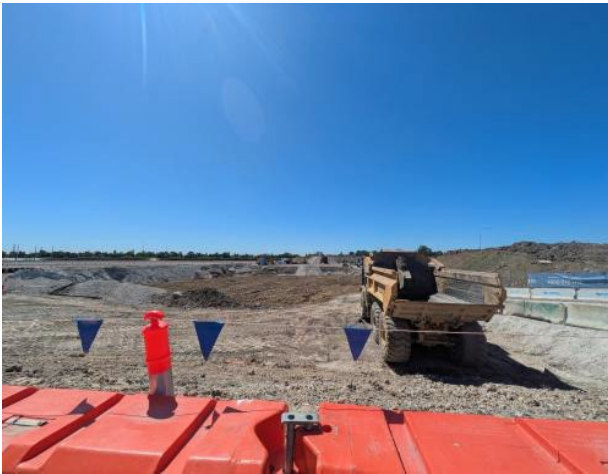
Figure 2.9 – Clyde MSF (West): Backfilling of previous site shed area.
