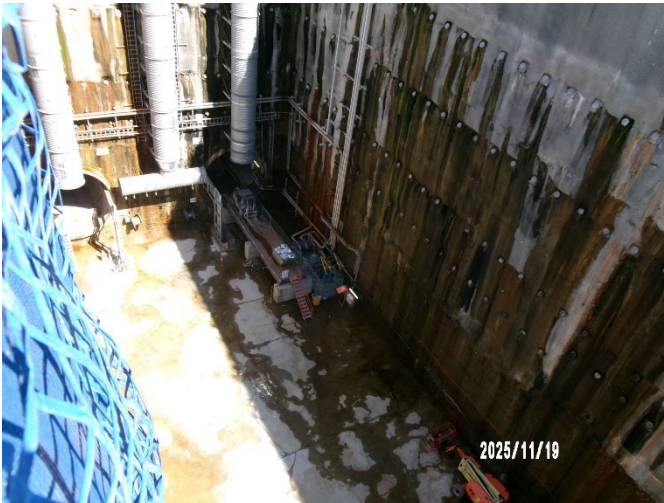
Figure 1.1 Station Box (The Bays) - Ongoing maintenance activities.
