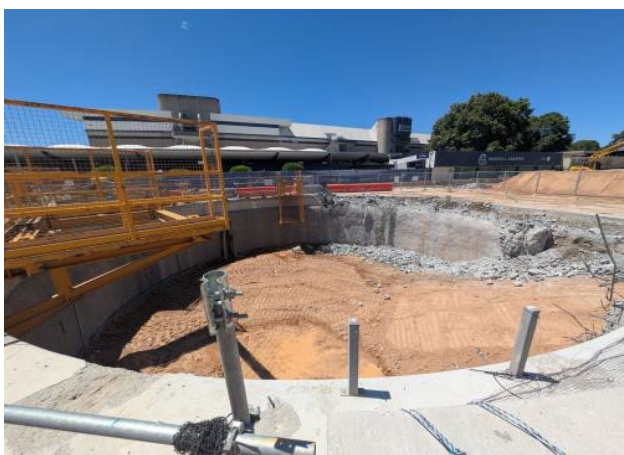
Figure 2.12 – Clyde Dive: Backfilling of shaft nearing completion.
