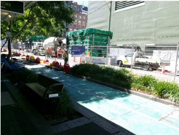
Figure 3.5 Pyrmont East: Set up of acoustic tents for concrete pumps.
