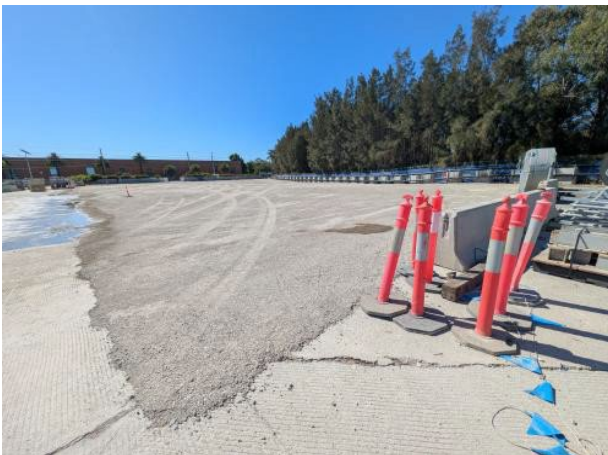
Figure 2.11 – Rosehill: Finishing works to handover Portion 2 Section continuing.
