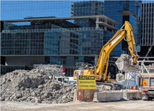
Figure 2.3 – Parramatta: Stockpiling and loadout of spoil.
