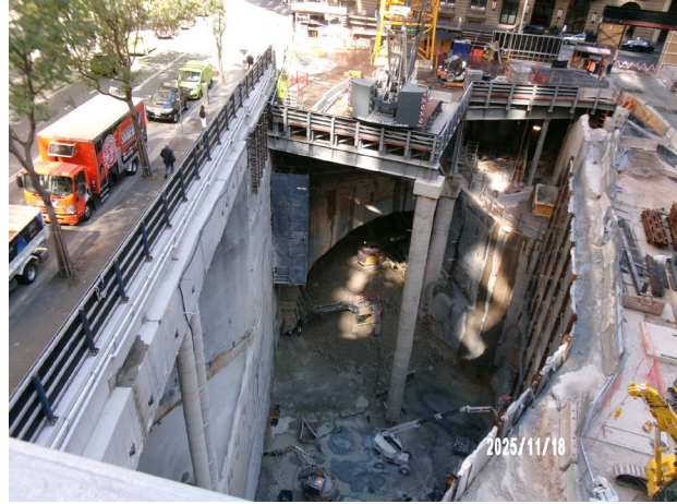
Figure 3.2 Hunter Street East: Completion of excavation adjacent Hunter Street.
