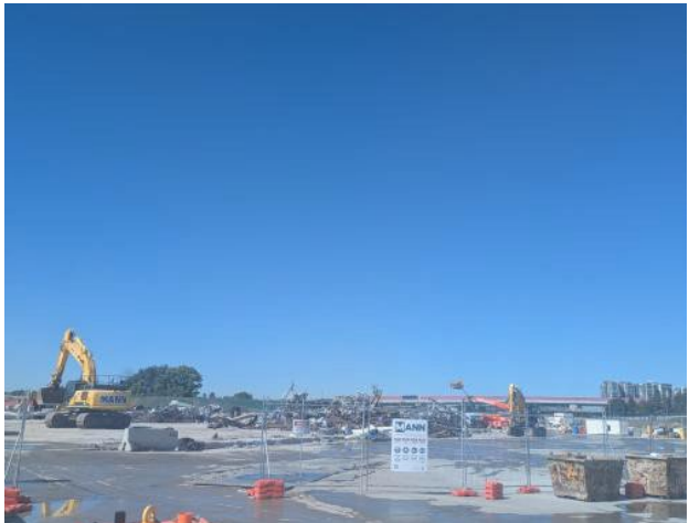
Figure 2.10 – Rosehill: Demolition of spoil shed completed.
