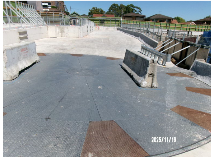
Figure 1.4 Western Shaft – no apparent works at the surface (Five Dock).
