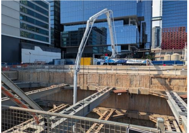
Figure 2.4 – Parramatta Eastern Station Box: Concrete boom pump set-up at surface level, for tunnel invert concrete pours.
