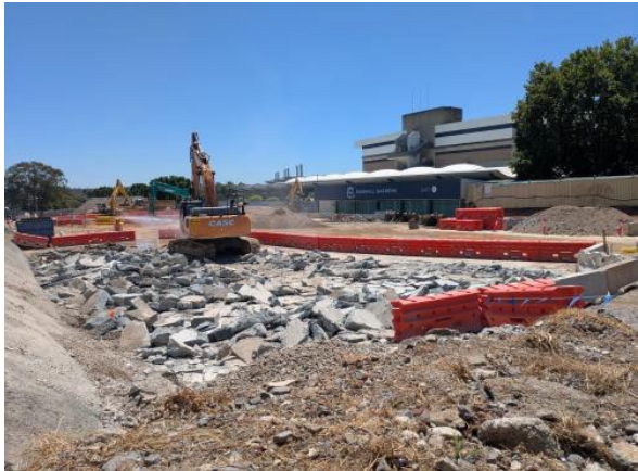
Figure 2.14 – Clyde Dive: Breaking of concrete with dust suppression observed.
