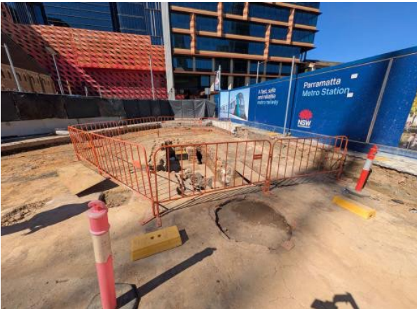
Figure 2.5 – Parramatta: Archaeological investigation and clearance works - Zone 10 (Macquarie Lane section).
