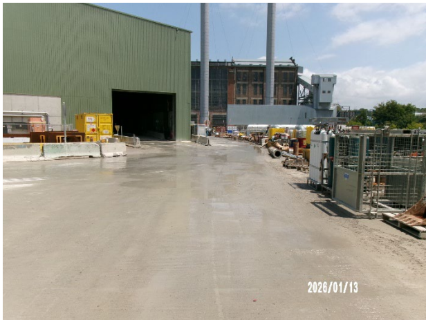
Figure 3.9 The Bays: Hardstand areas outside spoil shed.
