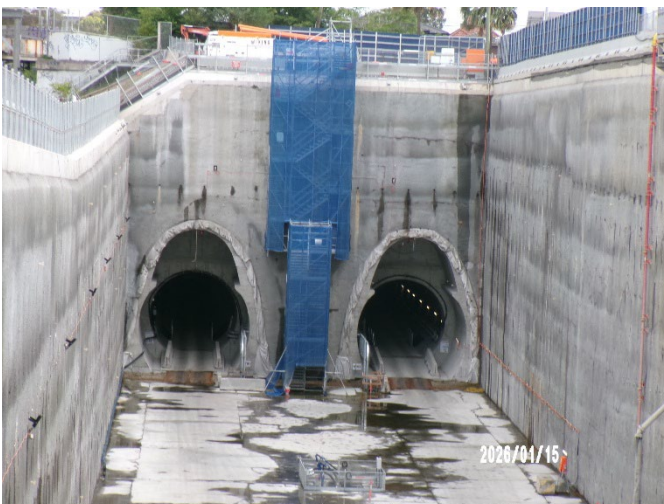
Figure 1.7 No works observed in the station box at North Strathfield (NS).
