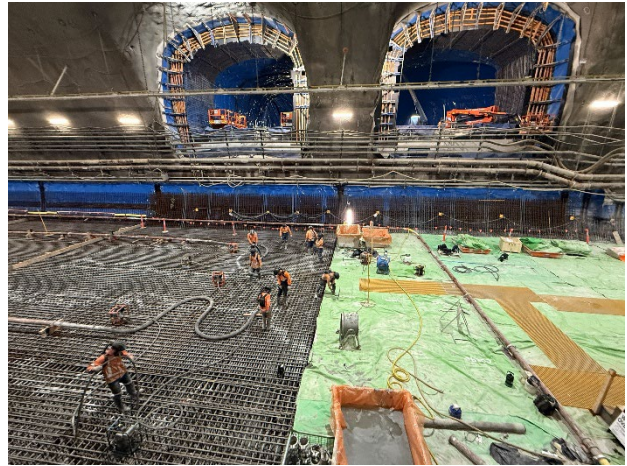
Figure 3.6 Pyrmont East: Invert pour near the service adits.
