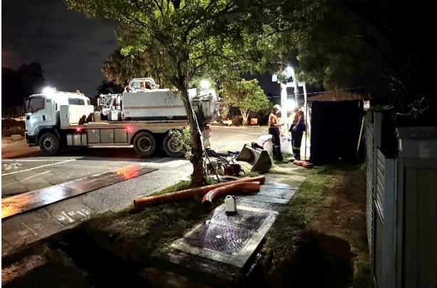
Figure 5.1 Sucker Truck reorientated with its next location of work, to have the truck noise further away from residences. Close to doubling the distance away from the receivers as compared to the initial positioning parallel to kerb line. Noise blankets also in place adjacent works.
