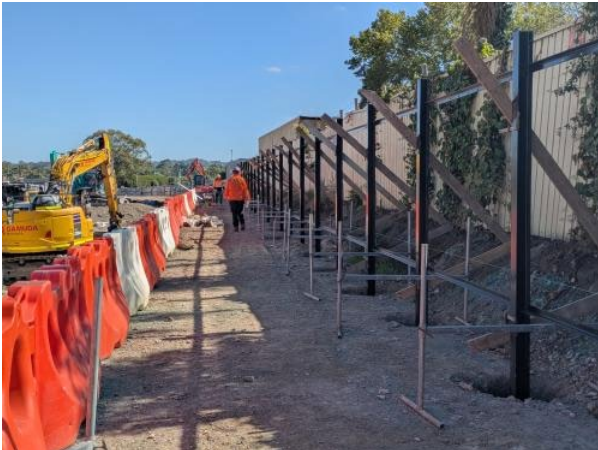
Figure 2.13– Clyde Dive: Fencing works along north-eastern section.
