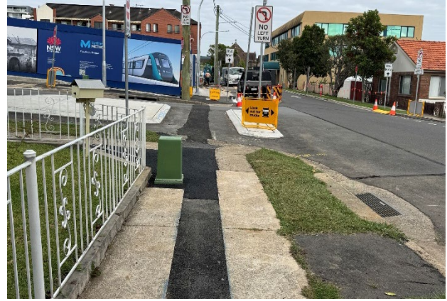
Figure 4.2 Completed all trenching on Second Ave and Waterview St.
