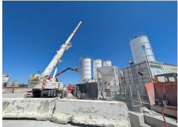
Figure 2.8 – Rosehill: Demobilisation of grout plant.
