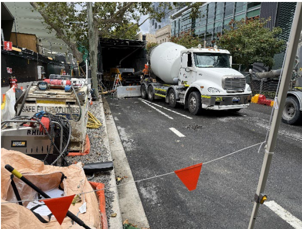
Figure 3.7 Pyrmont East: Concrete delivery on Union Street.
