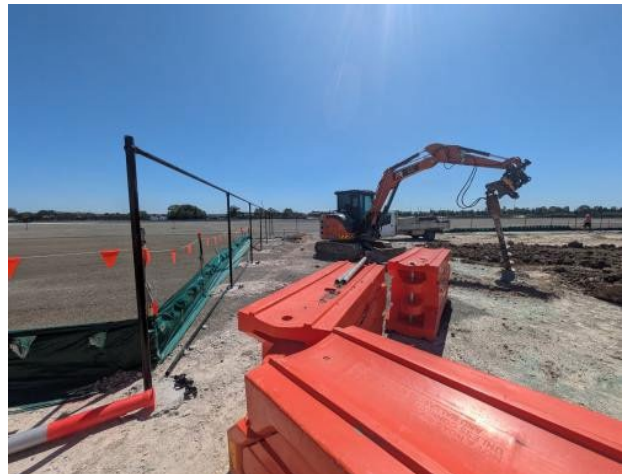
Figure 2.10 – Clyde MSF (West): Pedestrian fencing work commenced and continuing.
