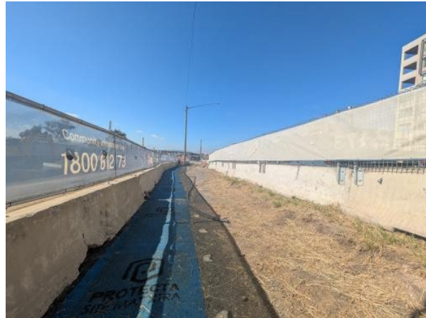
Figure 2.14 – Clyde Dive: Perimeter concrete barriers requiring JRD closure completed on 21 January 2026.
