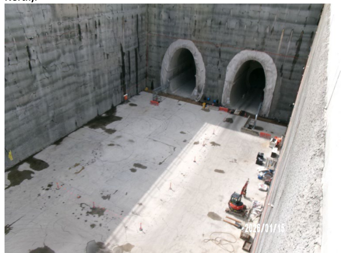
Figure 1.8 Station Box (SOP).
