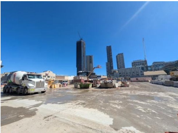
Figure 2.3 – Parramatta: Hardstand areas wet down.
