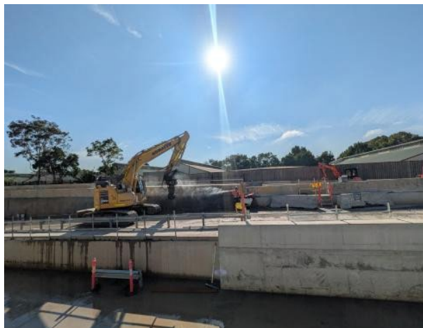
Figure 2.9 – Clyde Dive: Dust suppression observed for scabbling activity.
