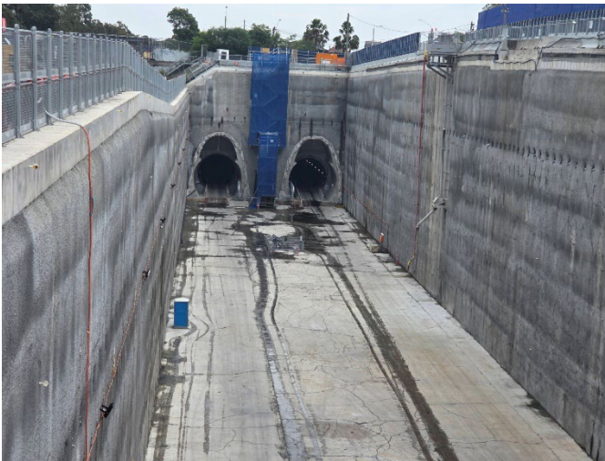
Figure 1.7 No works observed in the station box at North Strathfield (NS).
