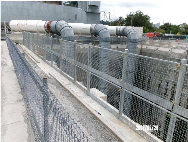
Figure 1.1 Station Box (The Bays) - Ongoing rectification and maintenance activities.
