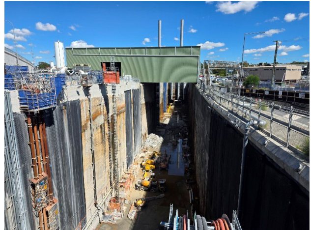
Figure 3.8 The Bays: Ongoing works in the base of the Station Box.
