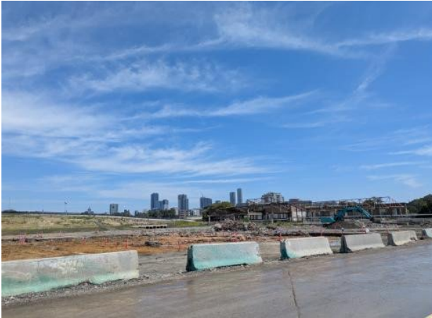
Figure 2.7 – Rosehill: Flood Basin Stage 2 works (no access).
