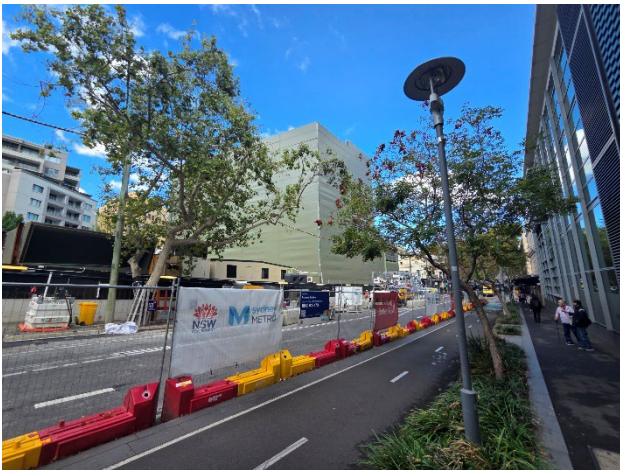
Figure 3.5 Pyrmont East: Concrete pumps removed from Union Street.
