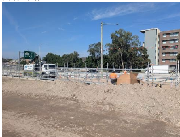
Figure 2.10 – Clyde Dive: Bulk earthworks and culvert works (Zone 3).
