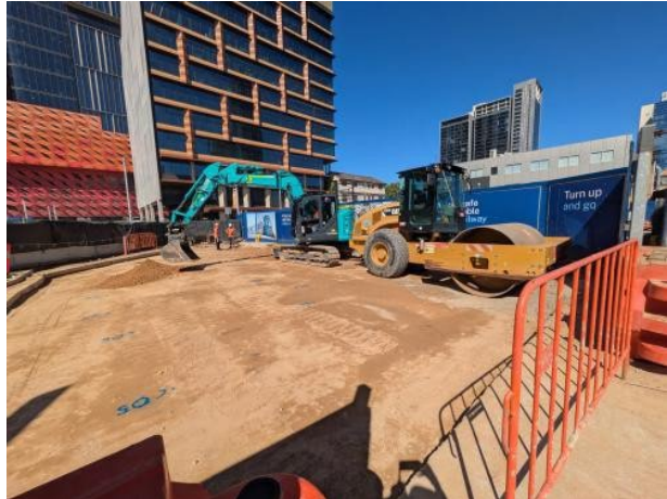
Figure 2.4 – Parramatta: Zone 10 - Macquarie Lane Section – Backfill and reinstatement.
