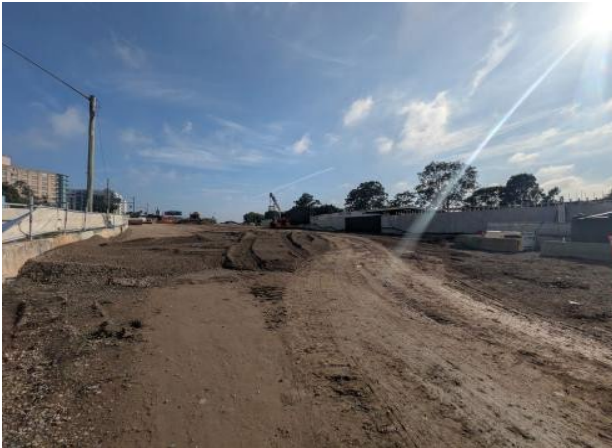
Figure 2.11 – Clyde Dive: Preparatory works underway for chipsealing surface (western section).
