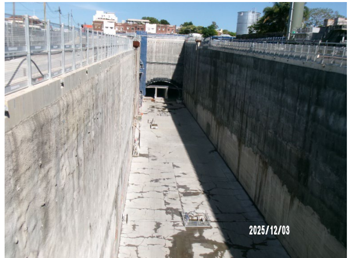
Figure 1.6 No visible activities occurring in the station box (Burwood North).
