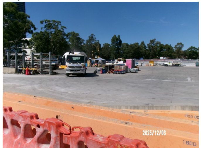
Figure 1.8 Ongoing use of workshop at the surface (SOP).
