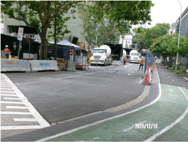
Figure 3.5 Pymont East: Concrete pumps in Union Street.
