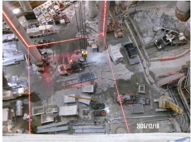
Figure 3.6 Pymont East: TBM support activities.
