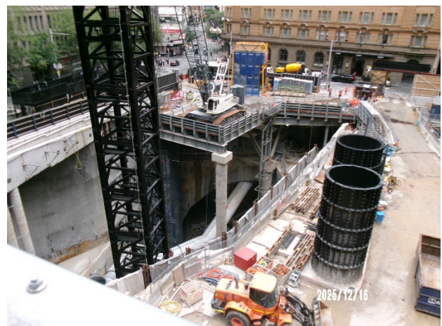
Figure 3.2 Hunter Street East: Installation of tower crane for TBM retrieval.
