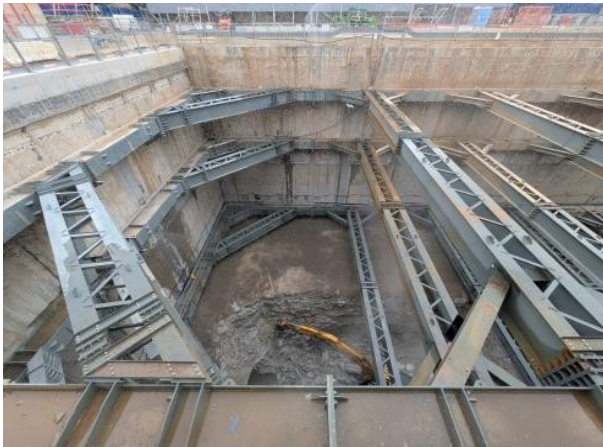
Figure 2.1- Parramatta Western Station Box: Hammering within box on Western end.
