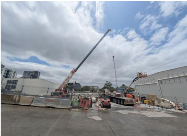
Figure 2.5 – Westmead: Cranage works - Surface Level.
