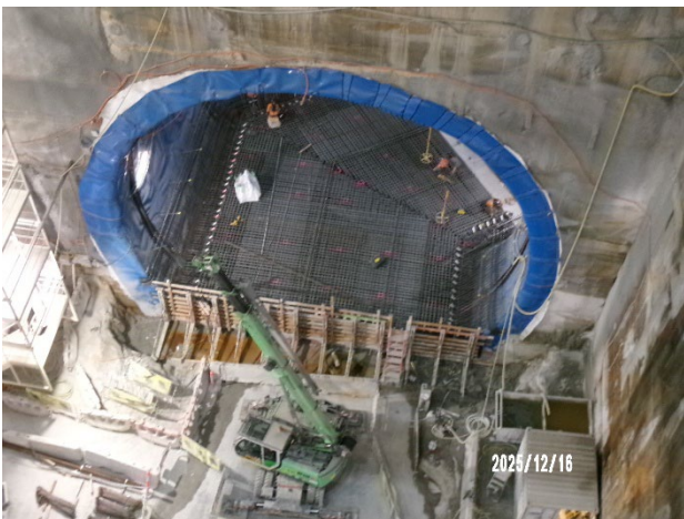
Figure 3.7 Pymont West: Service adit FRP works.
