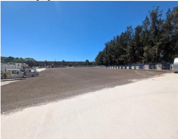
Figure 2.11 - Rosehill: Chipseal of section of Portion 2 completed.
