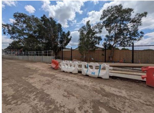
Figure 2.14 – Clyde Dive: Fencing works along section of eastern boundary.
