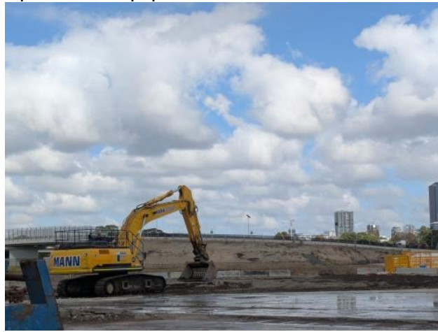
Figure 2.12 - Rosehill: Concrete removal for Flood Basin Stage 2 works commenced.
