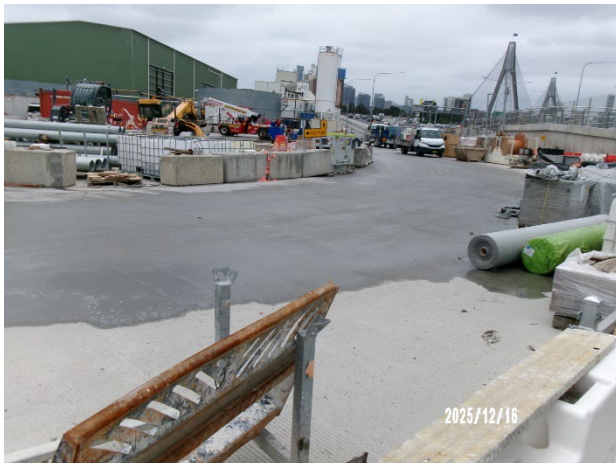
Figure 3.9 The Bays: Truck marshalling area.
