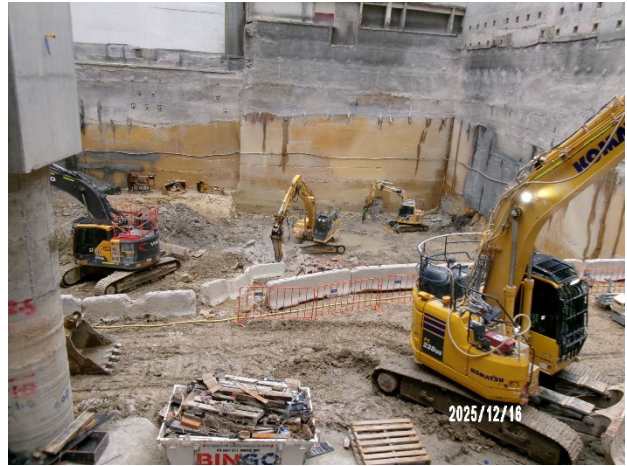
Figure 3.4 Hunter Street West: Ongoing excavation of the shaft.
