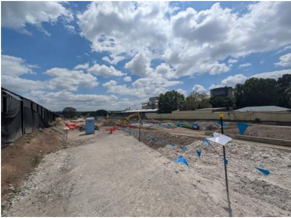
Figure 2.13– Clyde Dive: Earthworks in Zone 3 continuing.
