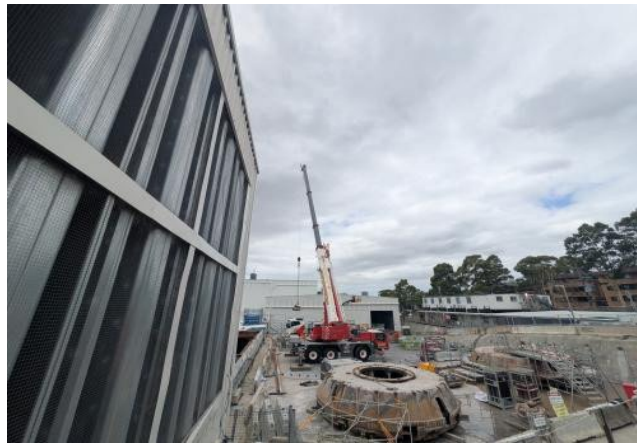
Figure 2.6 – Westmead: TBM cutter heads lifted to surface.
