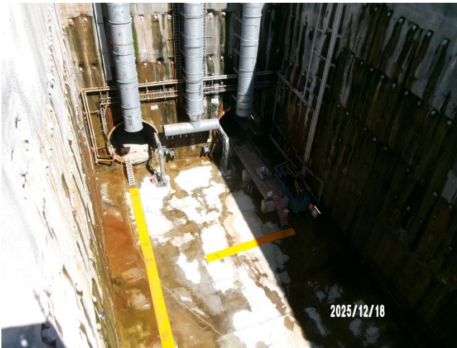
Figure 1.1 Station Box (The Bays) - Ongoing maintenance activities.
