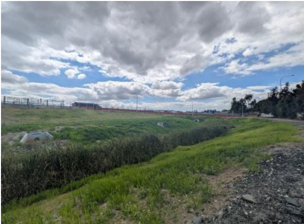
Figure 2.7 – Clyde MSF (West) – Grass take observed in previously hydromulched area.
