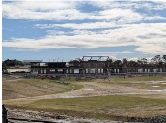
Figure 2.14 – Clyde MSF Site: Stage 1 of Flood Basin excavation and construction completed.
