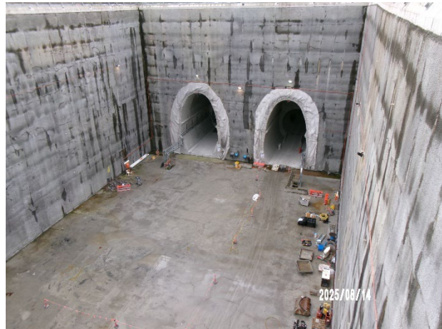
Figure 1.8 Access for maintenance works in the tunnel (SOP).
