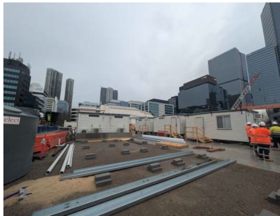
Figure 2.6 – Parramatta Site: Area 7 - site shed relocation works.
