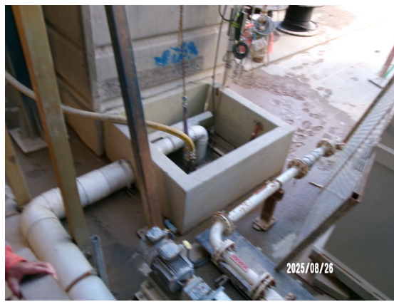
Figure 3.10 The Bays: Water management controls in place and operating.
