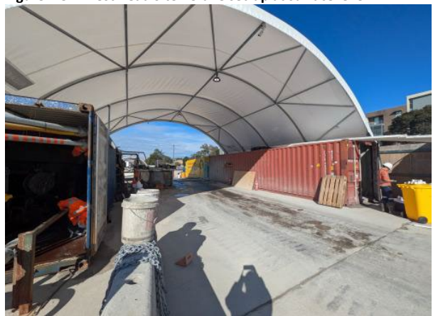
Figure 2.10 – Clyde Dive Site: Grouting Igloo - no concrete deliveries observed.
