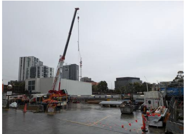
Figure 2.8 – Westmead Site: Crane set-up at surface level.
