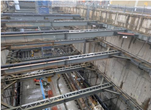
Figure 2.1- Parramatta Site: TBM 2 traversing station box.
