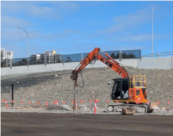
Figure 2.13 – Clyde MSF Site: Augering underway for fence post.
