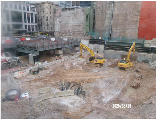
Figure 3.3 Hunter St West: Steel deck construction.
