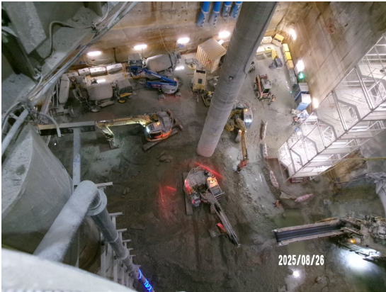
Figure 3.7 Pymont West: Load out of spoil ongoing.
