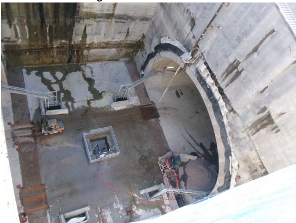
Figure 1.3 Eastern Shaft – works completed – ongoing repairs and maintenance activities (Five Dock).
