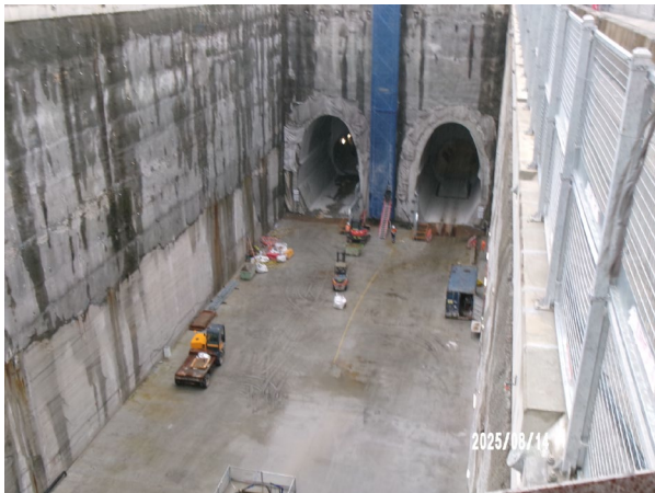
Figure 1.5 Ongoing maintenance in the nozzles (Burwood North).
