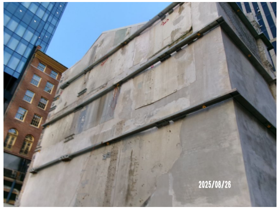
Figure 3.4 Hunter Street West: Strengthening works at Skinner's Hotel.
