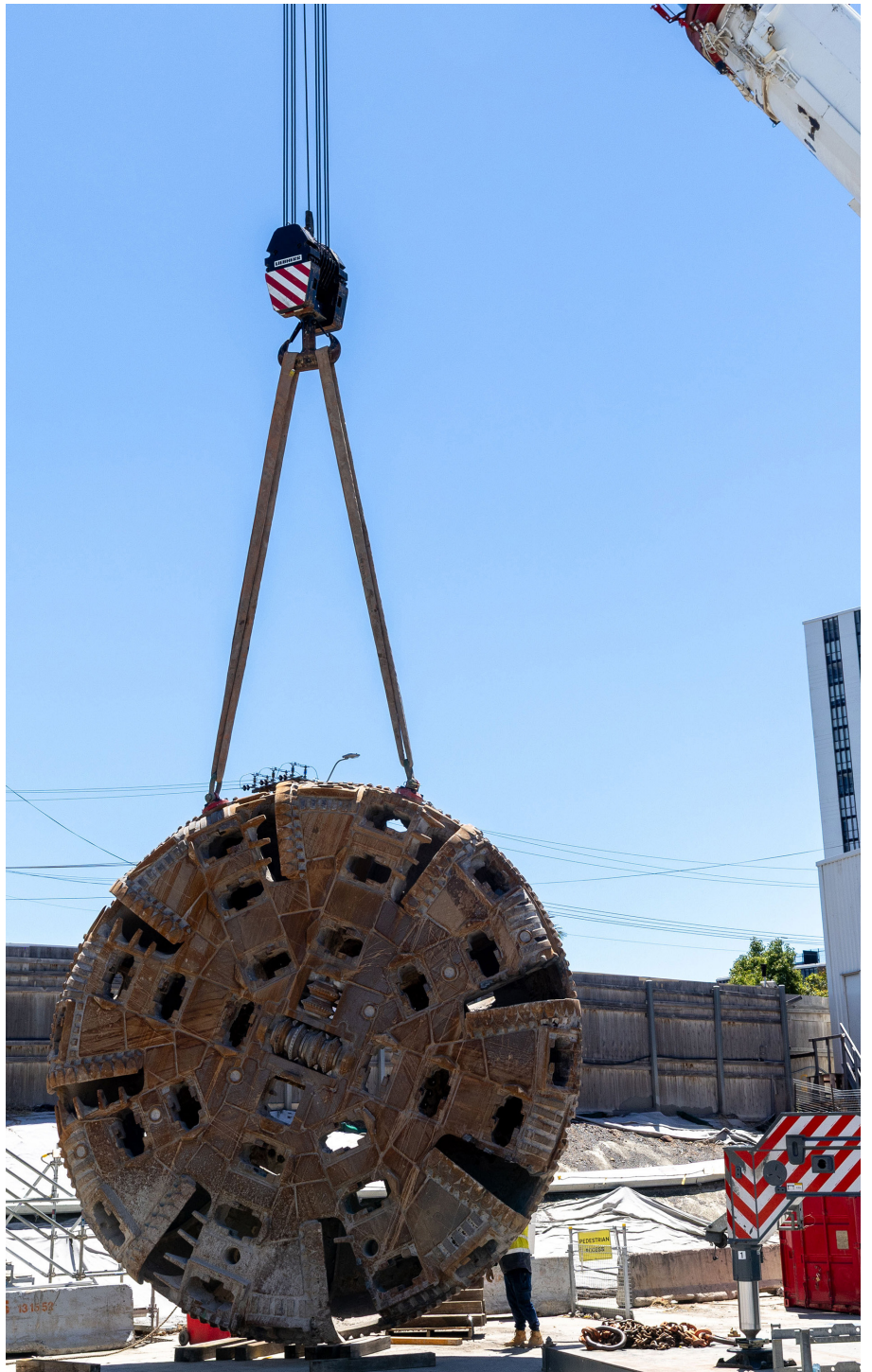
TBM Betty's cutterhead back on the surface.
