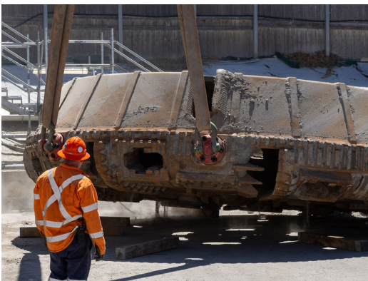
The cutterhead is lowered face-first to the ground.
