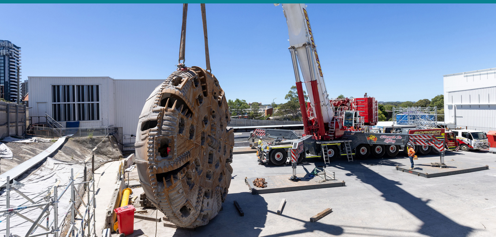
Tunnel boring machine (TBM) Betty's cutterhead, back on the surface at Westmead.
