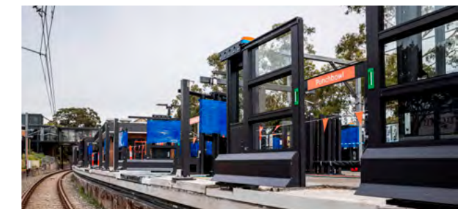
Image: Screen door installation on Punchbowl Station platforms.
