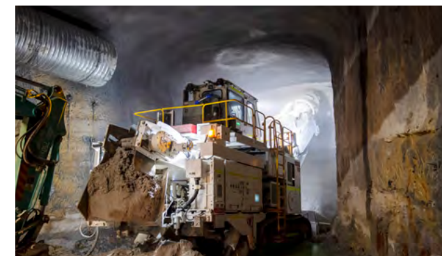
Image: Road header excavating tunnel at the Hunter Street Station site.
