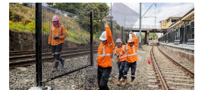
Image: Fencing installation along the boundary of the Southwest Metro corridor.
