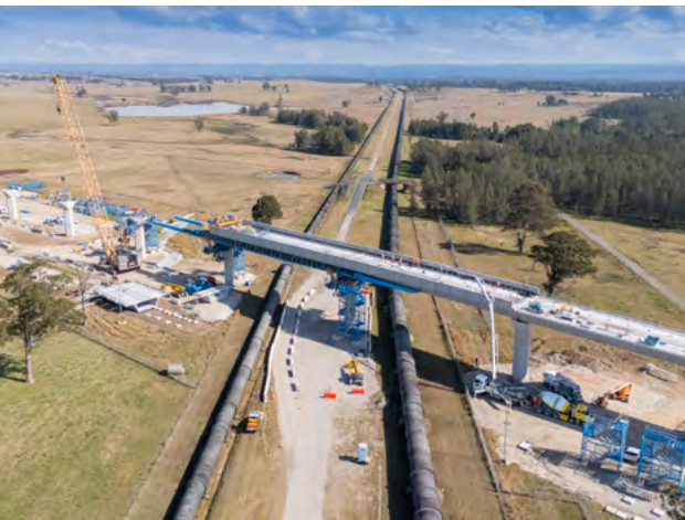
Image: View of the complex engineering technique used to place segments to form the viaduct over the Warragamba pipeline.
