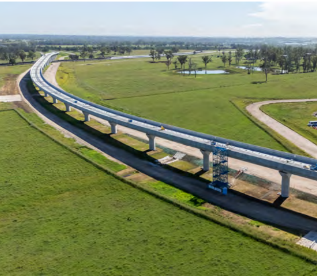
Image: An aerial view of the completed viaduct.
