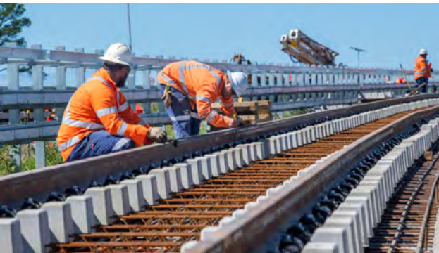
Image: Track laying work for the new Sydney Metro – Western Sydney Airport Line.
