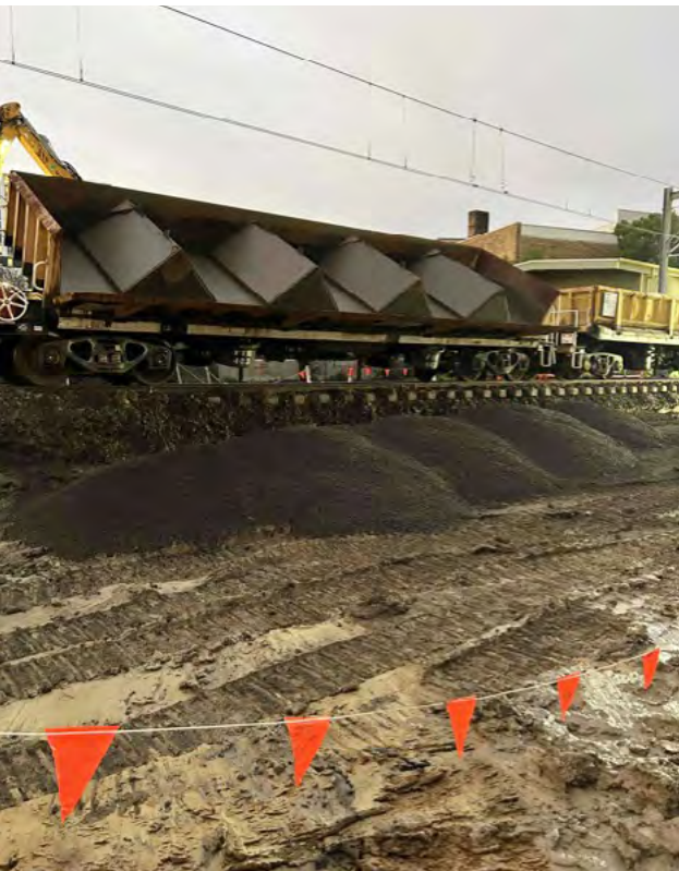
Image: Recycled ballast deposited onto Sydney Metro Southwest tracks.
