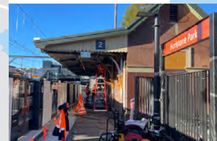
Hurlstone Park Station
