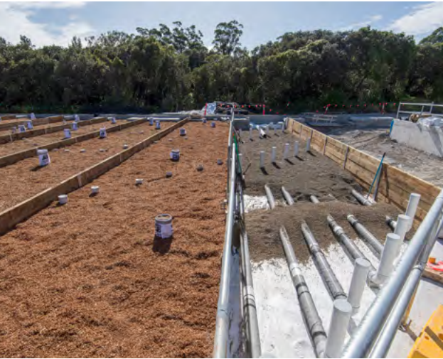
Images above: Bio Basin installation at the Clyde Maintenance Service Facility.
