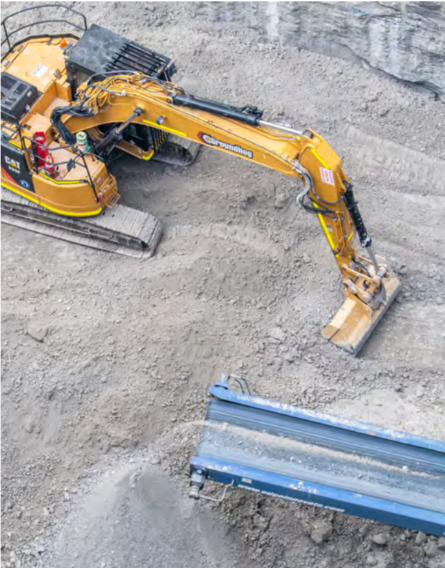
Image: Spoil being removed from the station box at The Bays Station site.
