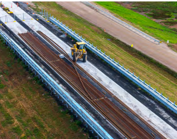
Image: Start of track laying at Luddenham.
