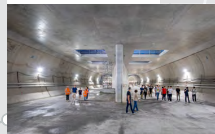
Burwood North Station
