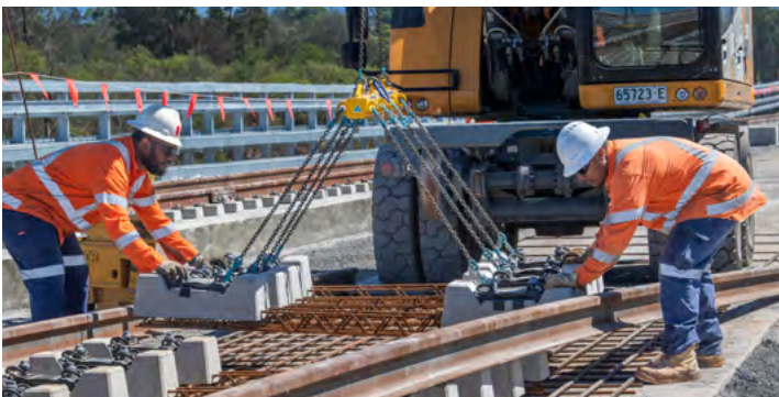
Image: Track works underway at Luddenham Station.
