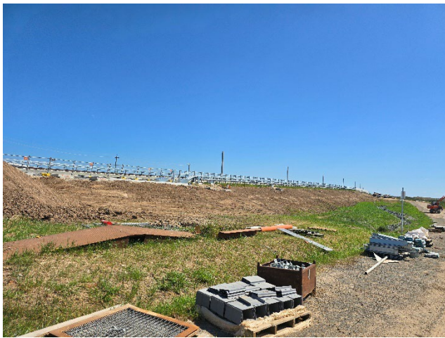
M12 to Elizabeth Dr – Laydown and CSR works. Re-establishment of batters to occur (discussed polymer with PLM).
