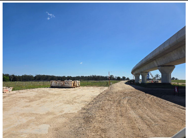
Water Pipeline to Luddenham Station – skip bins on stabilised pad with vegetation buffer to fenceline.
