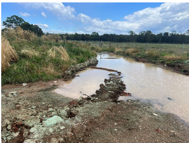
BSF – ESC to be checked at laydown boundary after dewatering.
