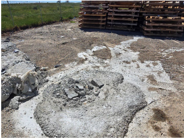
Luddenham to M12 – Concrete washout adjacent to M12.
