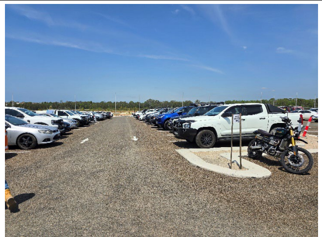
BRD – New car park construction completed.
