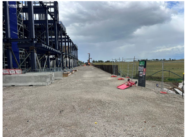
LUD – Sheet piling and structural steel work continued.
