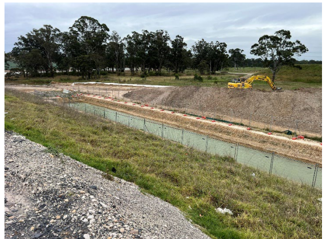
SMF – Topsoil amelioration stockpile and swale to be decommissioned.
