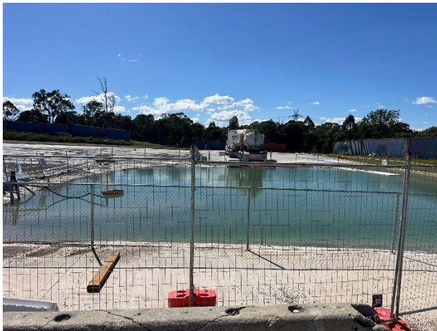
OHE – Dewatering of the concrete batch plant's sump was occurring with water being taken off-site for treatment.
