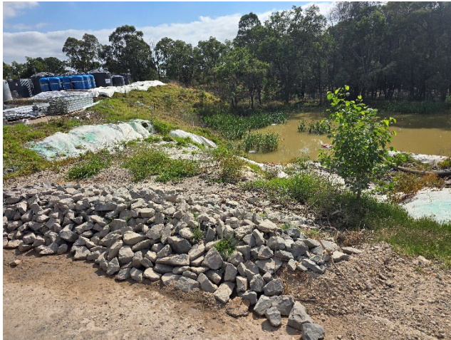
OHE – Rock check bund installed at refilling point adjacent to northern basin.
