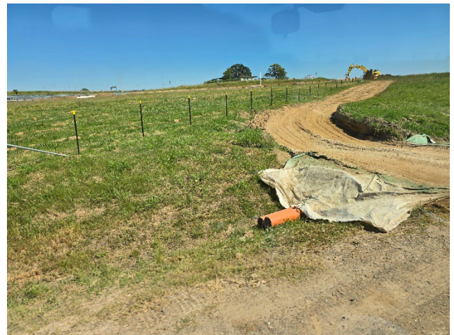
M12 to Elizabeth Dr – Swale crossing upgraded with drainage pipes, ESC on track to be monitored.
