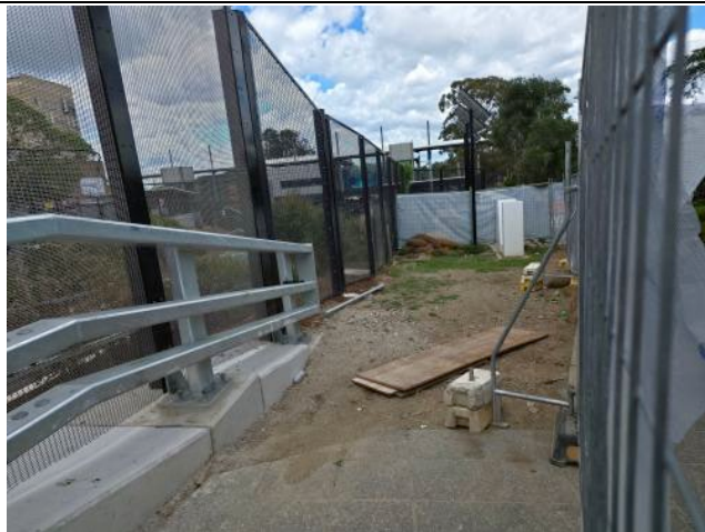
Figure 5 – Haldon St, Lakemba - Barrier installation complete, landscaping works being planned.
