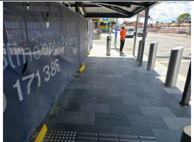
Figure 6 - Canterbury Road, Canterbury - Bollard installation complete, pavers have been installed and area has been reinstated.
