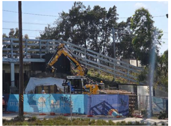
Figure 2 – Ness Ave, Dulwich Hill - Overhead crash beam installation works ongoing. Piling in progress.
