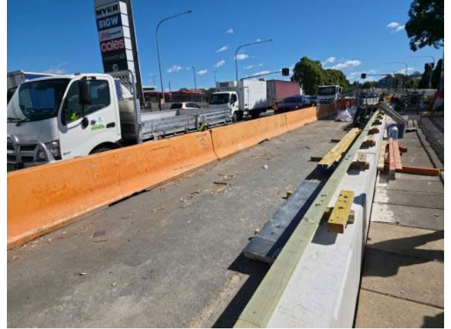
Figure 2 – Stacey St, Bankstown – South Terrace - Bridge Strengthening works completed at this site. Demobilisation of plant/equipment complete.
