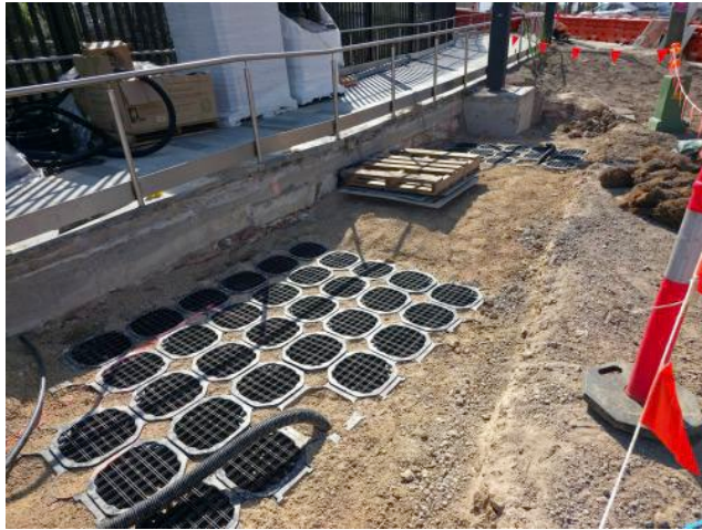
Figure 1 – Dulwich Hill Station – Plaza landscaping works and paving ongoing.
