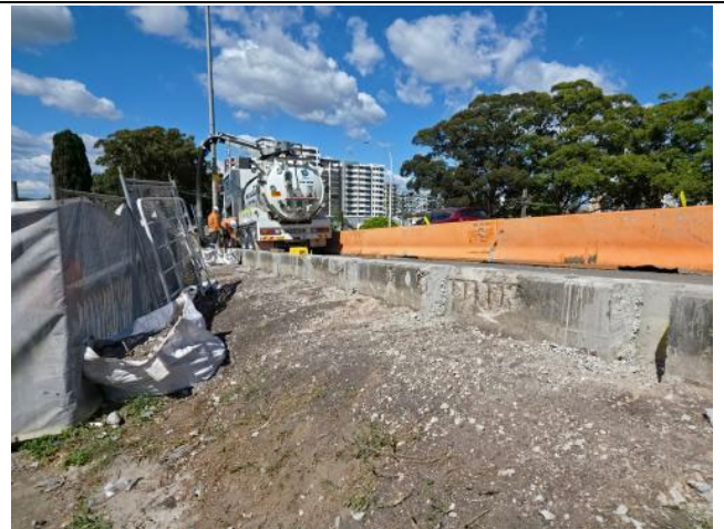
Figure 4 – Stacey St – Stage 2 – Light pole electrical cable related works ongoing. Non-destructive utility search ongoing.
