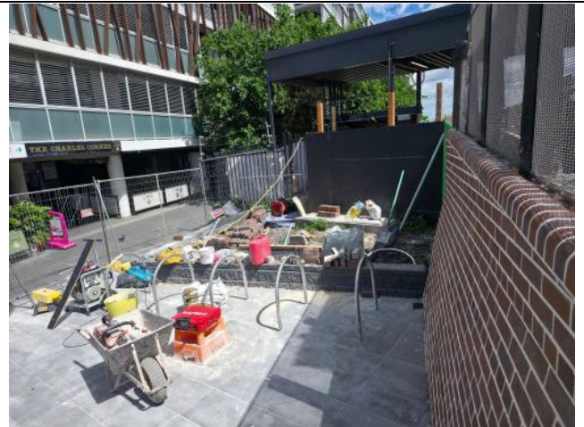
Figure 7 - Canterbury Station Plaza - Retaining wall installation complete. Landscaping works to follow in the coming weeks.
