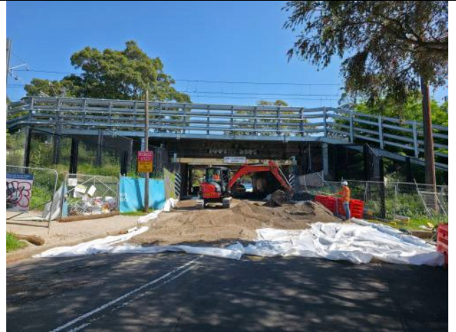
Figure 4 – Foord Ave, Hurlstone Park - Traffic control established, overhead crash beam installation works commenced.
