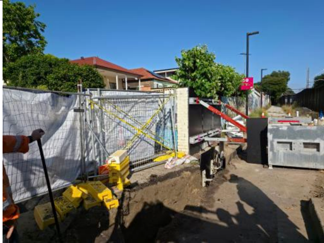
Figure 3 – Riverdale Ave, Marrickville - Sewer vent relocation works ongoing.
