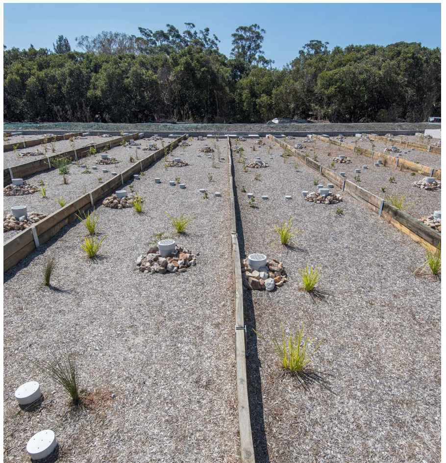
Smart, sustainable design: vegetation beginning to grow in the bio-basin
