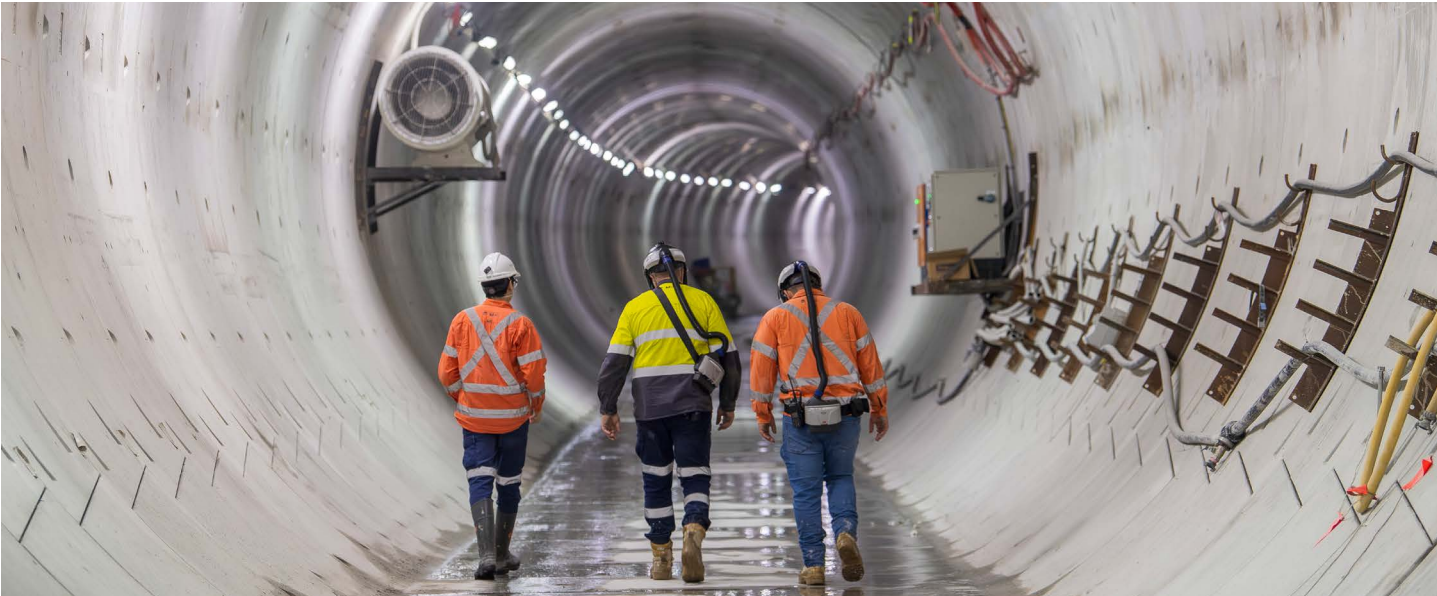
A look inside one of the finished service tunnels.
