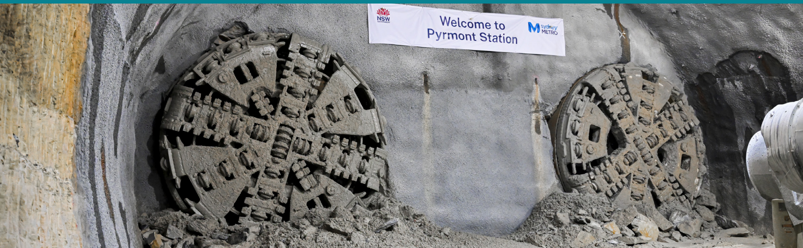
Tunnel boring machines (TBMs) Ruby and Jessie successfully broke through into the Pyrmont cavern in August.
