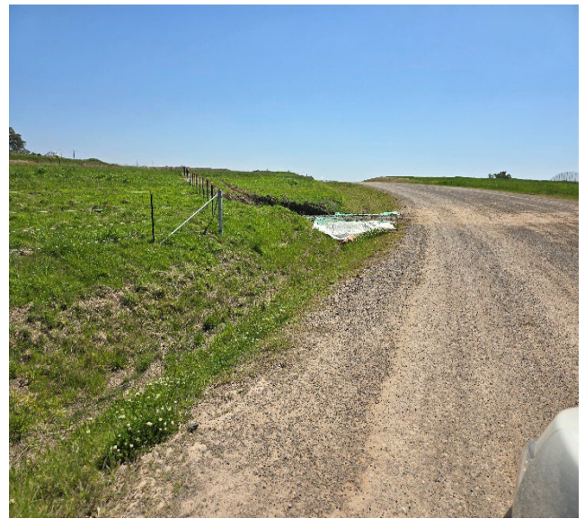
M12 to Elizabeth Dr – Swale crossing installed with pipes and Geofab. New tracks to be monitored for erosion.
