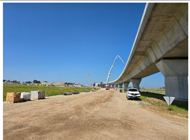
Water Pipeline to Luddenham Station – Concrete pump to viaduct and laydown on stabilised areas.
