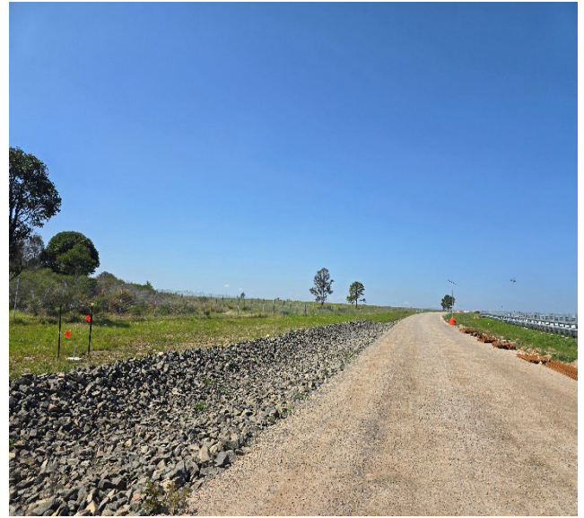
Luddenham to M12 – Haule road with speed bumps, laydown on stabilised area and rock-lined swale maintained.
