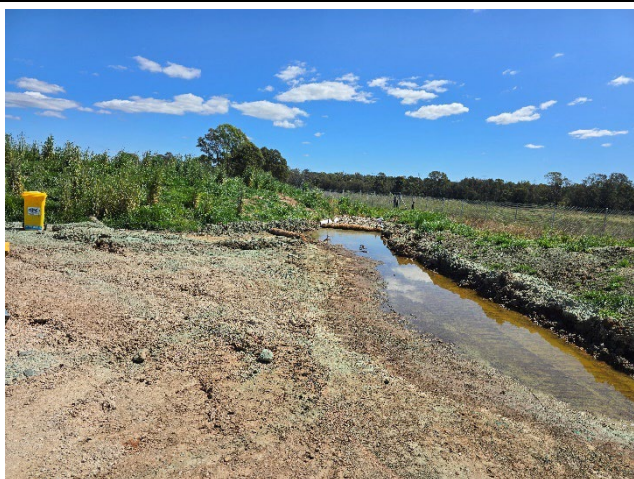
BSF – ESC had been maintained and sediment had been removed from the stabilised exit pad.
