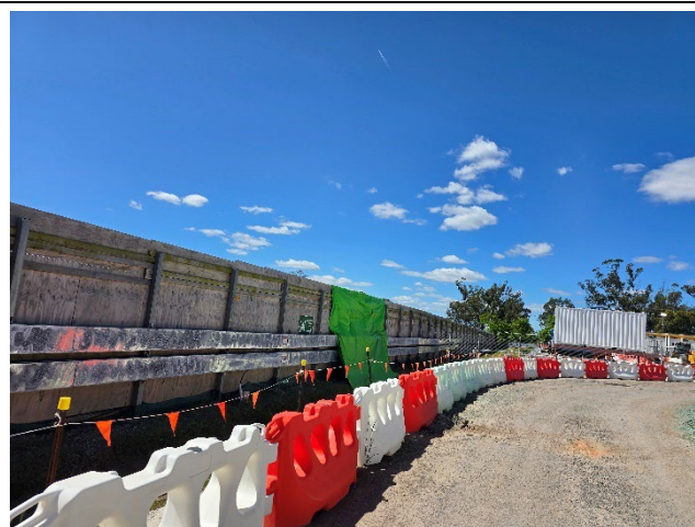
BSF – Additional noise mitigation to reduce reflected noise from the ventilation fan.
